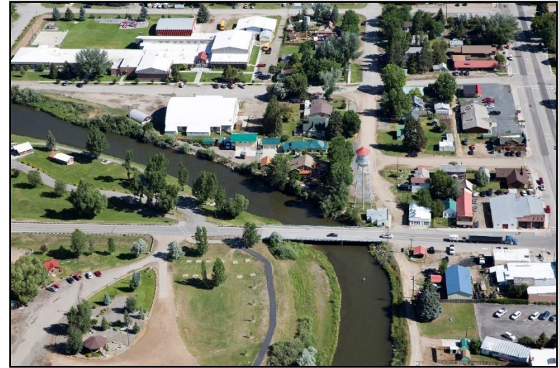
Figure 99. Highway 41 bridge in Dillon at river mile 2.2, July 21, 2016. (Kestrel)
