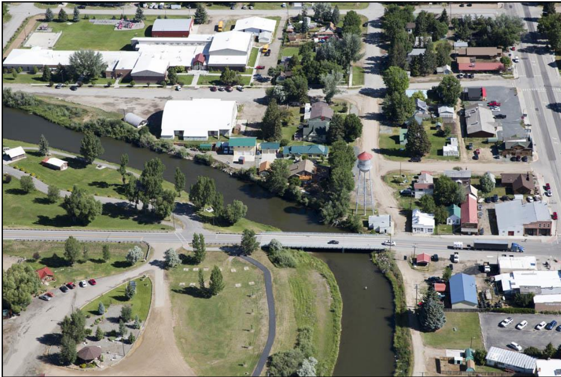
Figure 71. View downstream showing the Beaverhead River in Twin Bridges. (Kestrel)
