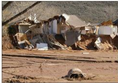
Figure 4. Photos from a 2005 flood in Saint George Utah, where homes several feet above the mapped floodplain were destroyed by channel migration ( www.Utahfloodrelief.com ).
