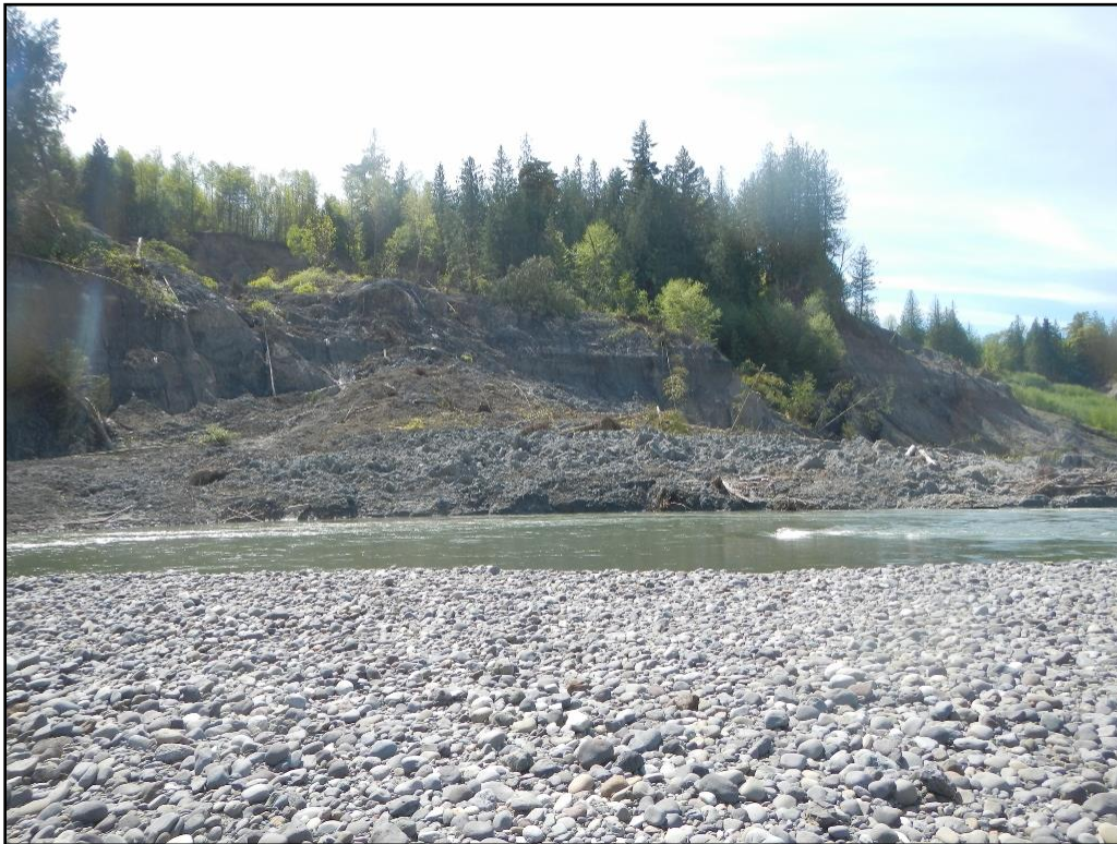
Figure 9. Hillslope failure on Nooksack River near Bellingham Washington on February 21, 2014.
