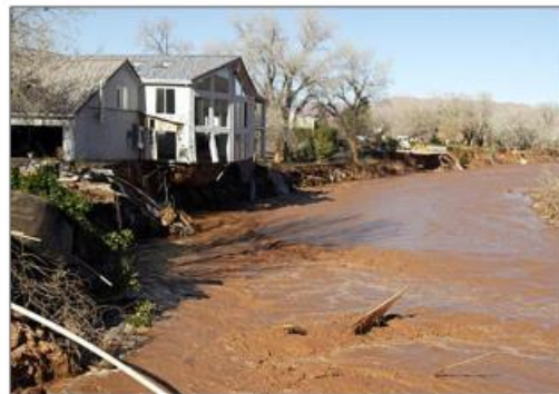
Figure 4. Photos from a 2005 flood in Saint George Utah, where homes several feet above the mapped floodplain were destroyed by channel migration ( www.Utahfloodrelief.com ).
