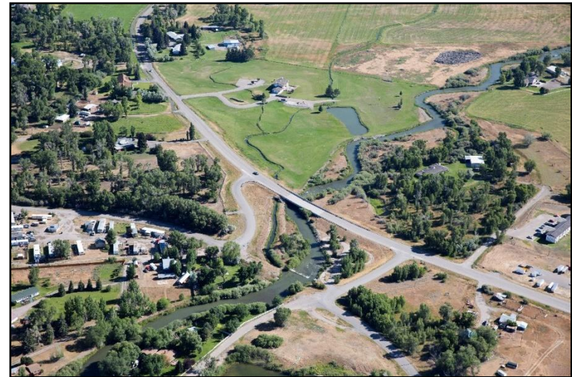
Figure 91. Highway 91 bridge at river mile 53.1, July 21, 2016. (Kestrel)
