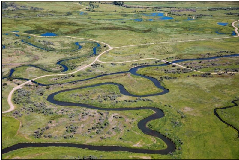
Figure 98. Private bridge at river mile 8.7, July 21, 2016. (Kestrel)
