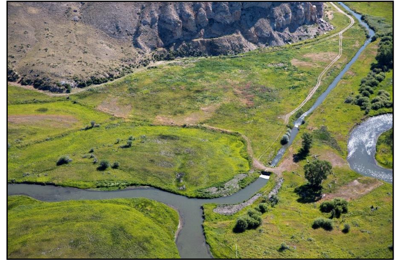
Figure 110. Co-op Ditch Diversion at RM 29.2 (Beaverhead Rock), July 21, 2016 (Kestrel).
