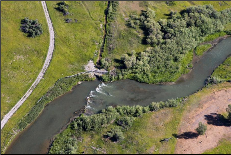
Figure 104. Diversion at RM 46.2 July 21, 2016 (Kestrel).
