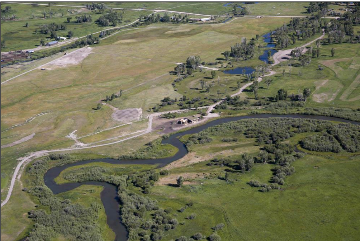
Figure 54. View north showing new home and ponds in historic channel trace that connected the Beaverhead River to Albers Slough. (Kestrel)
