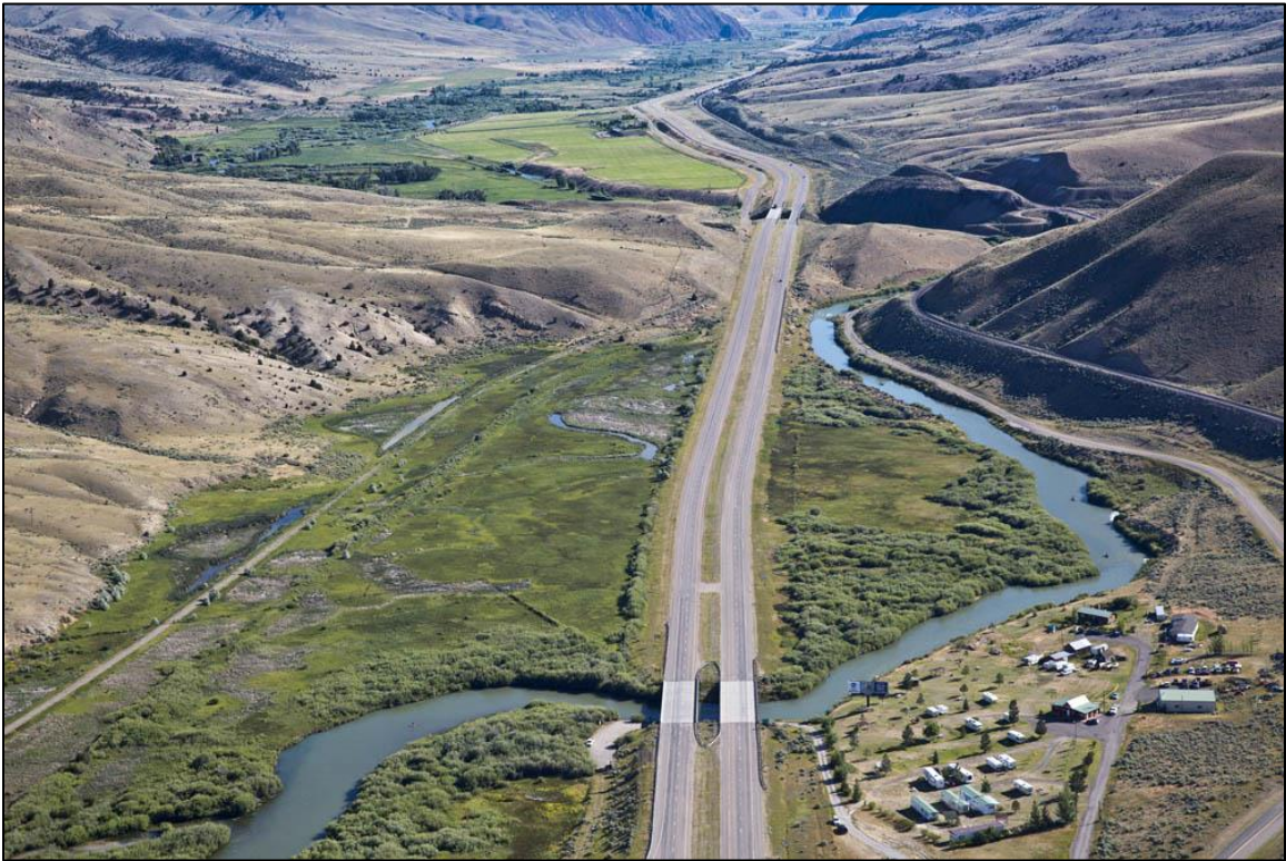
Figure 15. View downstream from near Clark Canyon Dam showing large a landslide deflecting the Beaverhead River to the east at High Bridge (Kestrel).
