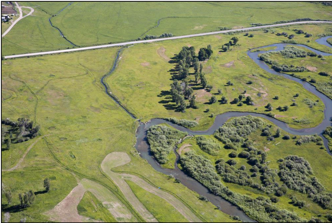
Figure 55. View downstream at RM 43.6 showing diversion structure at risk of abandonment by bendway cutoff. (Kestrel)
