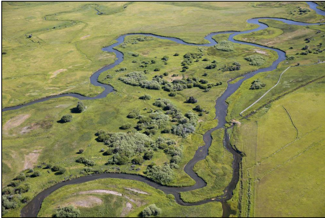
Figure 59. View downstream showing area of 1979-2013 avulsion RM 35.8; new channel is to left. (Kestrel)
