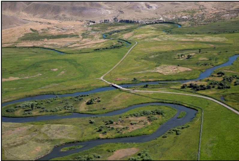
Figure 94. Diamond O Ranch bridge at river mile 33.1, with Albers Slough at the top of the image, July 21, 2016. (Kestrel)
