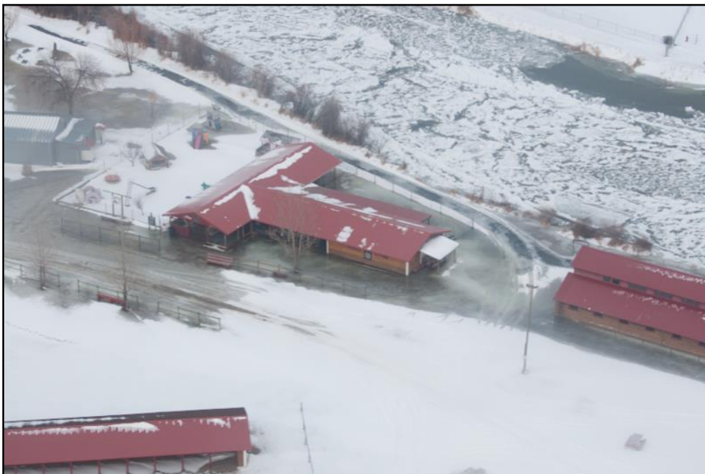
Figure 8. Ice jam and flooding at Twin Bridges, MT, January 4, 2011. (Madison County, MT Office of Emergency Management).
