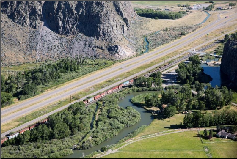
Figure 81. Barretts Park bridge at river mile 68.0, July 21, 2016. (Kestrel)
