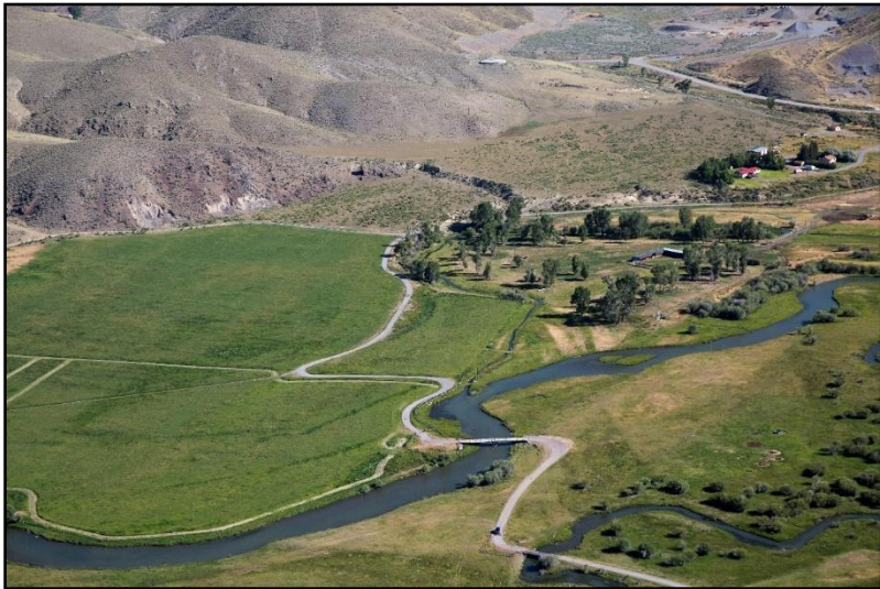
Figure 86. Private road bridge at river mile 57.1, July 21, 2016. (Kestrel)
