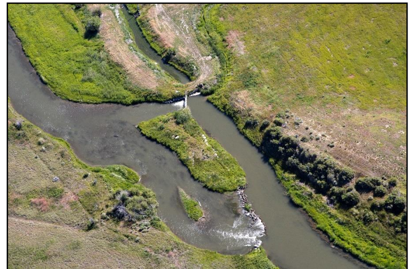
Figure 111. Diversion at RM 26.4, July 21, 2016 (Kestrel).
