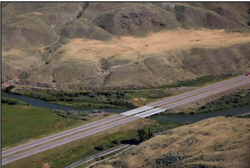
Figure 78. Interstate 15 (5 th crossing) at river mile 70.9, July 21, 2016. (Kestrel)
