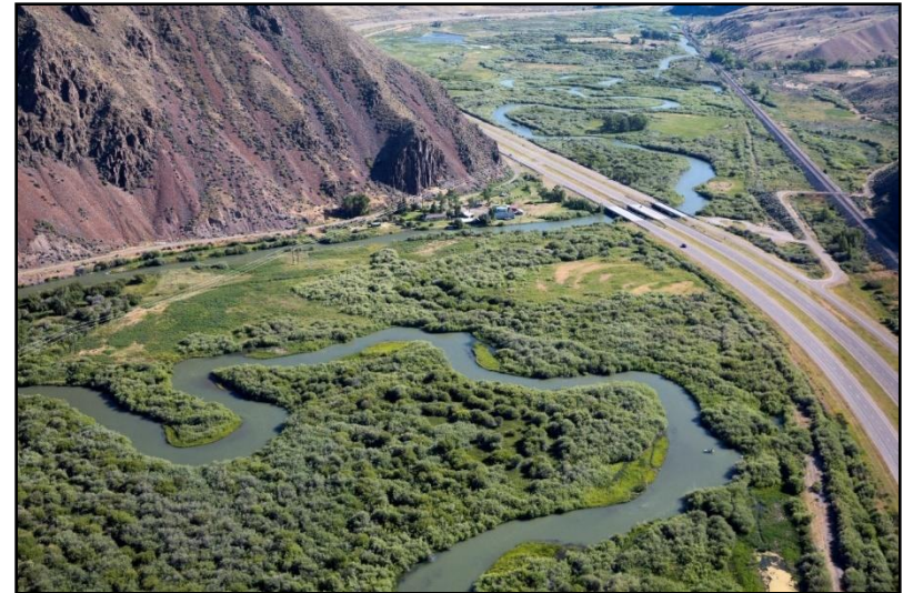
Figure 76. Interstate 15 (3 rd crossing) and High Road at river mile 75.4, July 21, 2016. (Kestrel)
