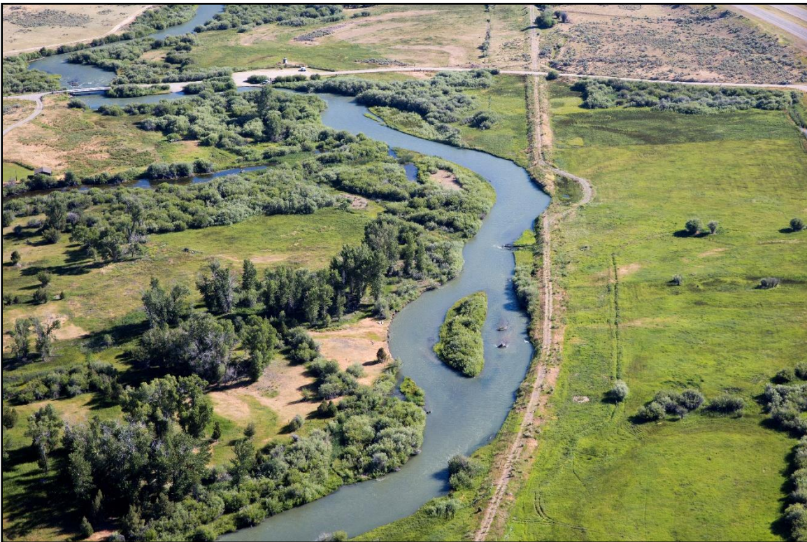
Figure 25. A historic rail grade in Clark Canyon showing a breach in the abandoned rail grade, July 12, 2016. (Kestrel)
