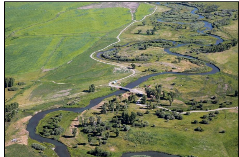
Figure 92. Private bridge at river mile 45.4, July 21, 2016. (Kestrel)
