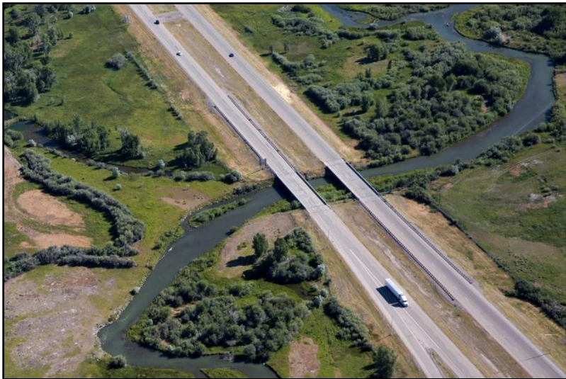
Figure 89. Interstate 15 (7 th crossing) at river mile 54.1, July 21, 2016. (Kestrel)
