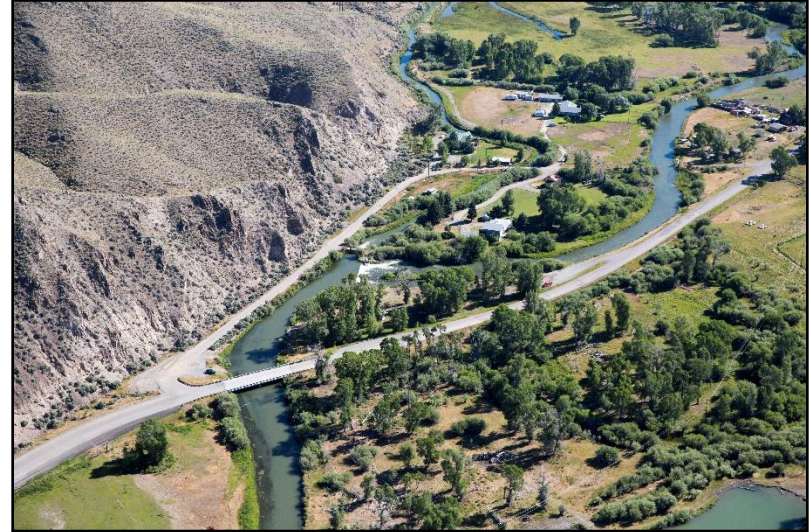
Figure 102. Smith Rebich Ditch Diversion at RM 55.6, July 21, 2016 (Kestrel).
