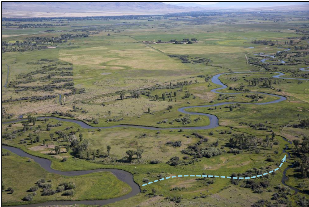
Figure 62. View downstream showing potential avulsion path through abandoned channel (right foreground), RM 17.7. (Kestrel)
