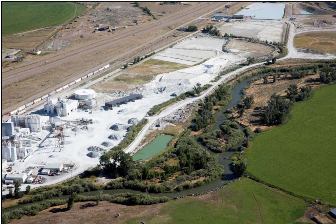
Figure 46. View downstream (north) showing channel confinement between Barrett Talc Plant and armored irrigated fields. (Kestrel)
