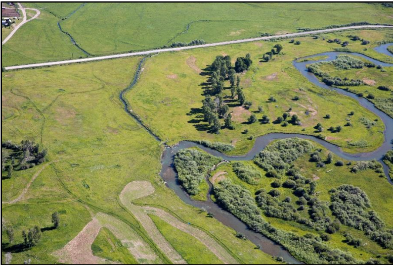
Figure 105. Diversion at RM 43.6, July 21, 2016 (Kestrel).
