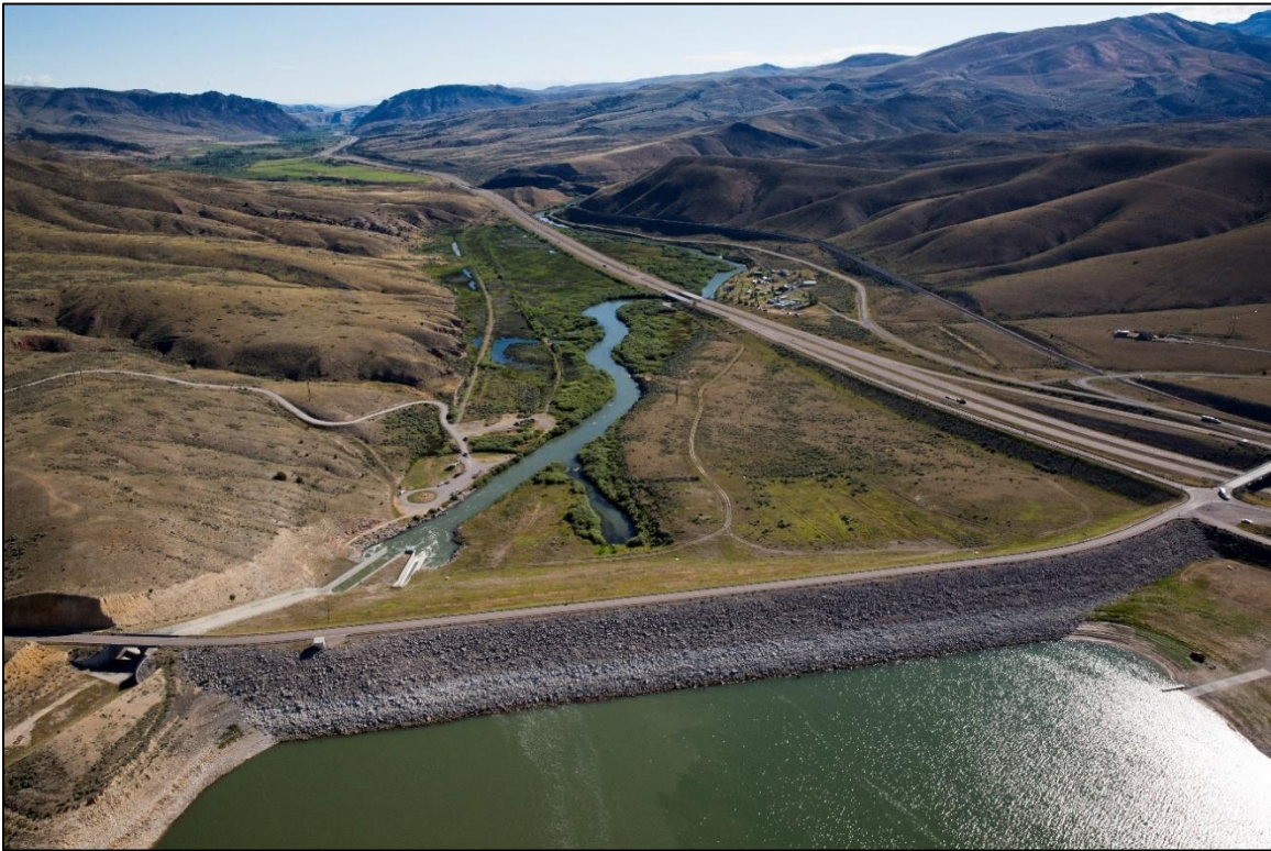
Figure 20. View downstream over Clark Canyon Dam, Montana. (Kestrel).
