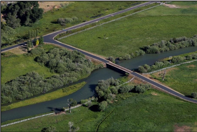
Figure 74. Hennaberry Road bridge (south) at river mile 80.4, July 21, 2016. (Kestrel)
