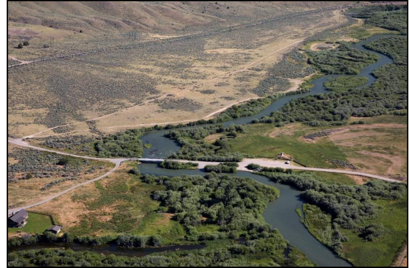
Figure 75. Hennaberry Road bridge (north) at river mile 77.3, July 21, 2016. (Kestrel)
