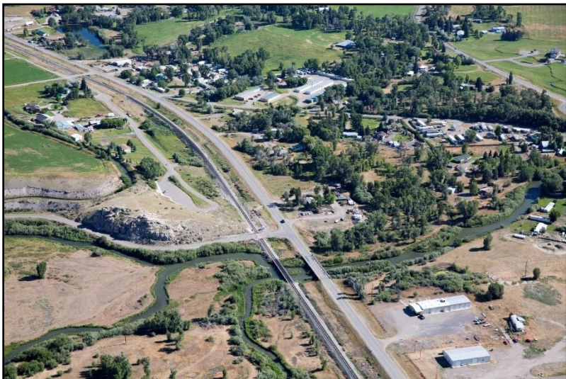
Figure 90. Union Pacific railroad and Highway 91 cross the Beaverhead River at river mile 53.5, July 21, 2016. (Kestrel)
