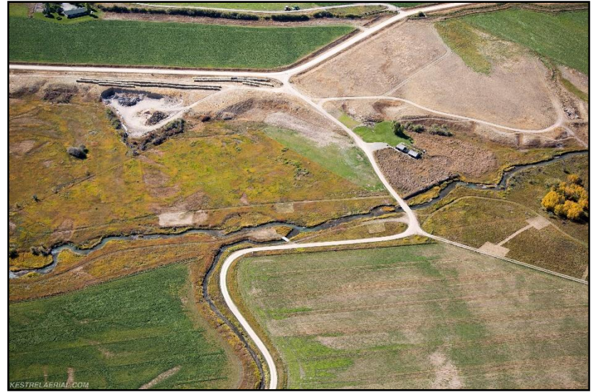
Figure 35. Farm bridge on Clear Creek RM 1.2 on September 29, 2017. (Kestrel)
