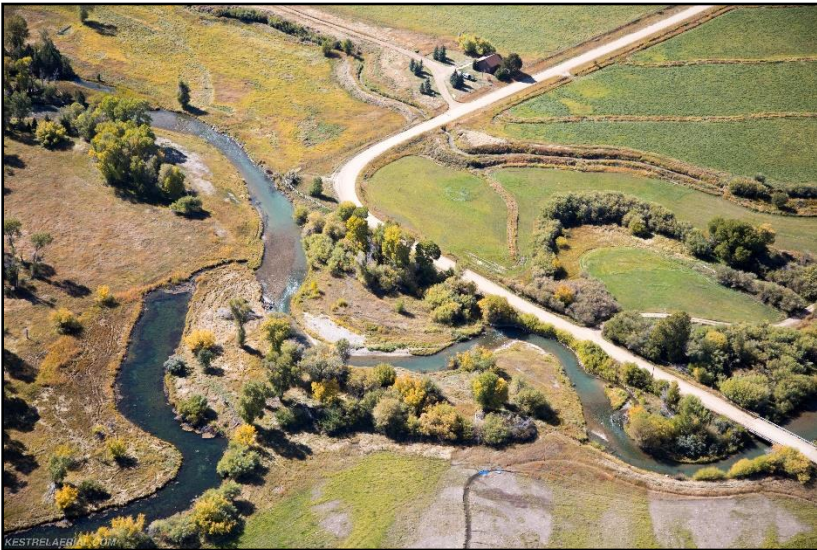
Figure 26. Judy Lane bridge on September 29, 2017. (Kestrel)
