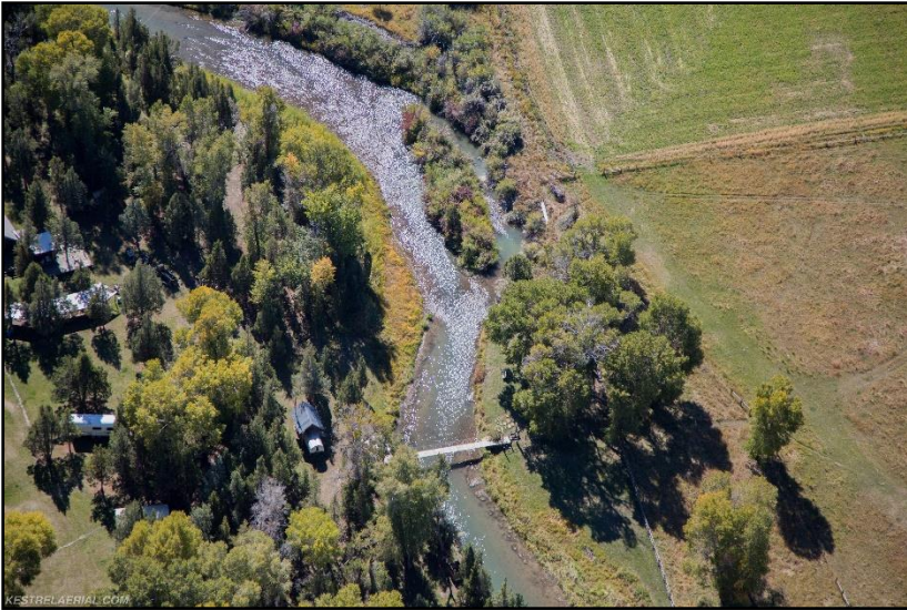
Figure 25. Private bridge at RM 50.5 on September 29, 2017. (Kestrel)
