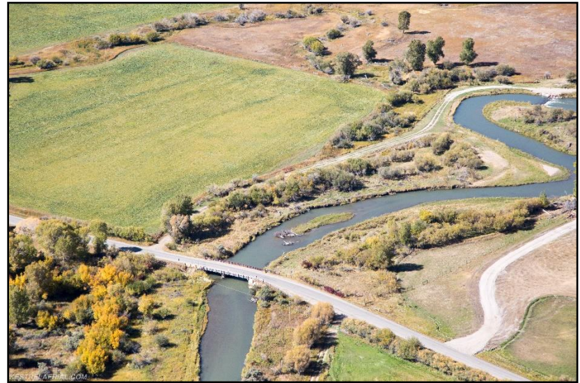
Figure 40. Seyler Lane bridge on September 29, 2017. (Kestrel)
