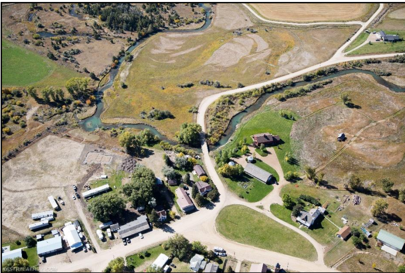
Figure 34. Ruby River Drive bridge on September 29, 2017. (Kestrel)
