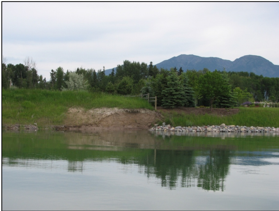
Figure 52. Boulder armor and local erosion, Flathead River.
