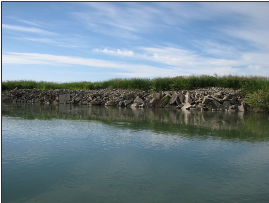
Figure 50. Typical concrete rubble revetment, Flathead River.
