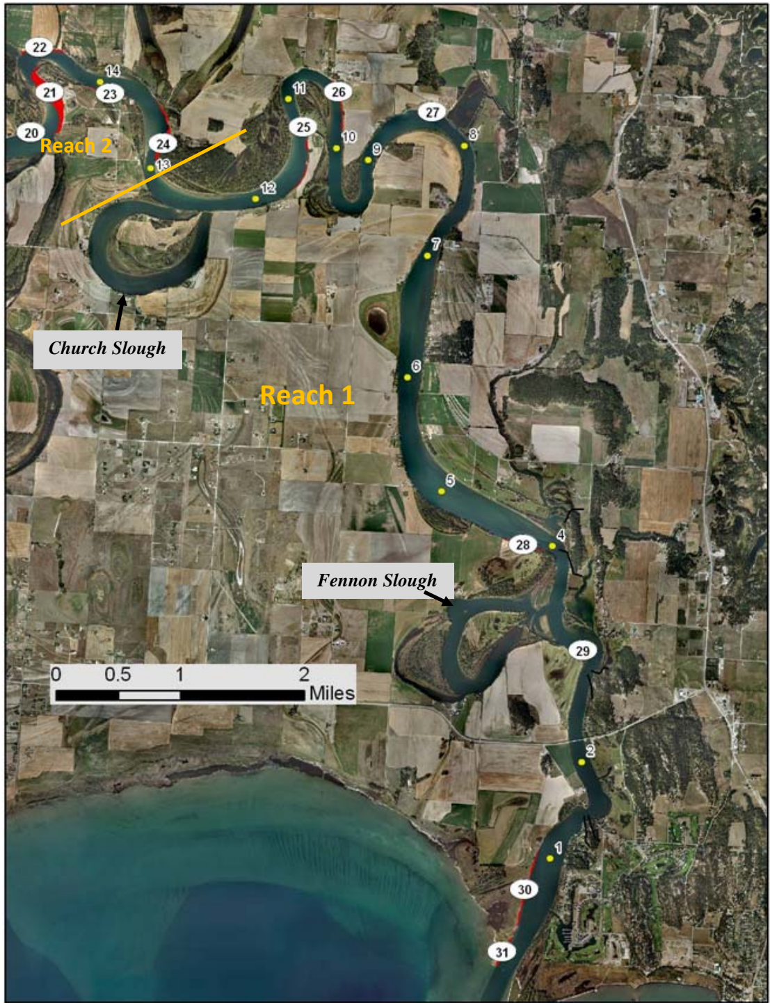
Figure 22. 2009 air photo of Reach 1, showing numbered erosion sites used in CMZ analysis.
