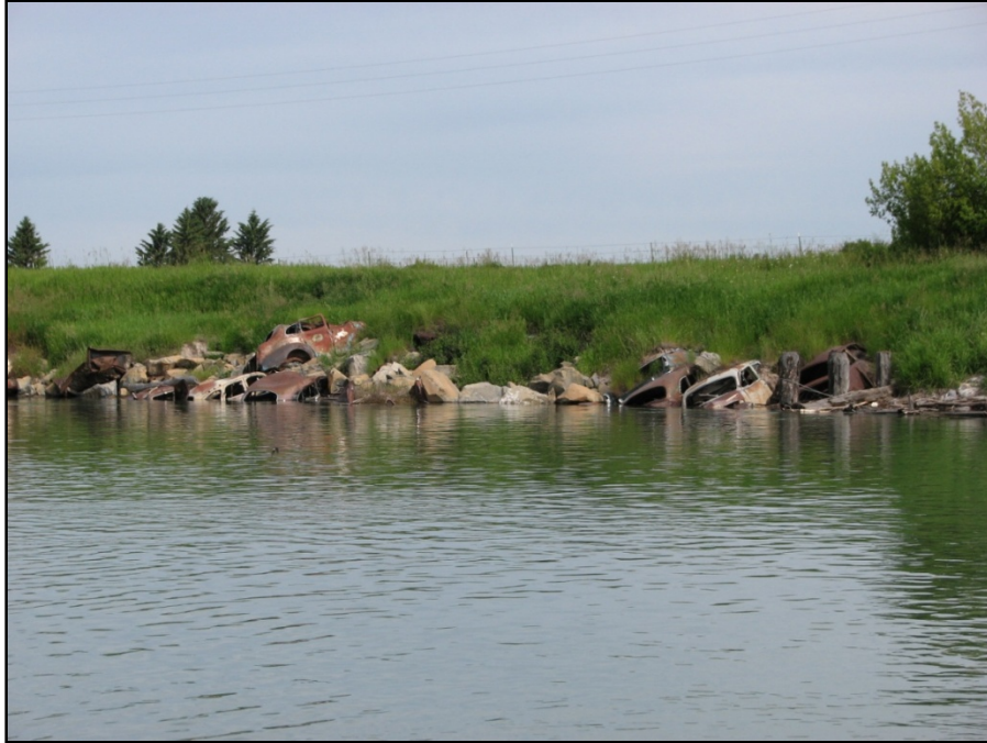
Figure 51. Rock riprap reinforcement over older car body revetment.
