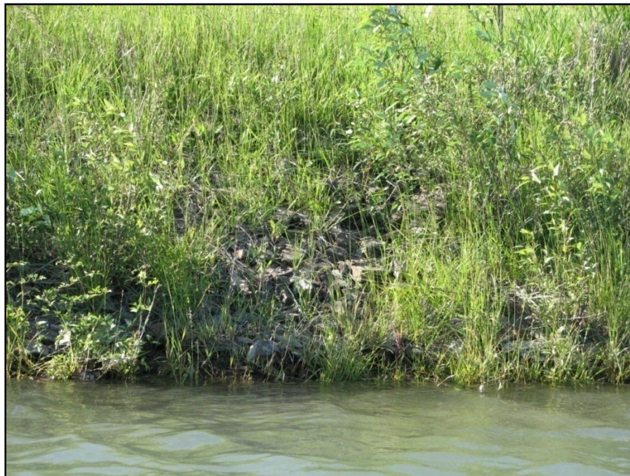
Figure 48. Quarried rock revetment obscured by vegetation, Flathead River.
