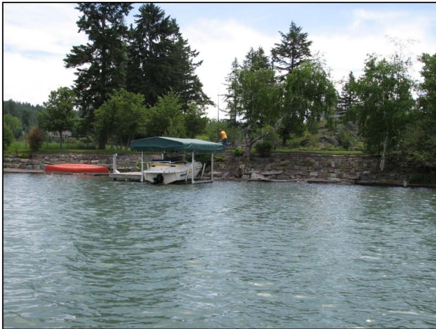
Figure 54. Stone wall revetment, Flathead River.
