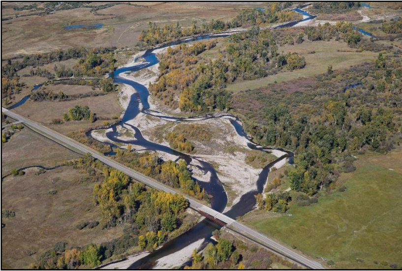
Figure 84. Dry Creek Road bridge on September 26, 2016. (Kestrel)
