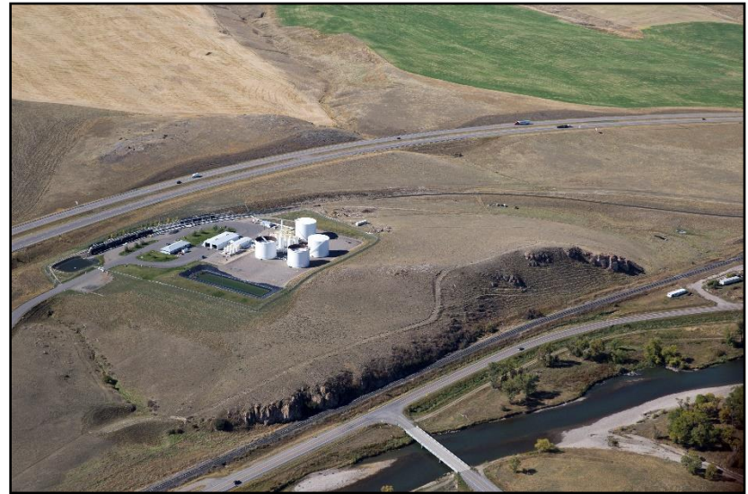
Figure 87. Logan Trident Road bridge on September 26, 2016. (Kestrel)
