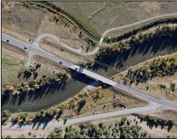
Figure 76. Hwy 191 bridge on September 26, 2016. (Kestrel)
