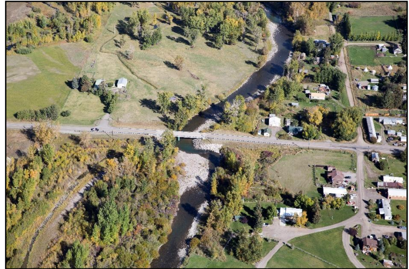
Figure 78. Gateway South Road (east span) bridge on September 26, 2016. (Kestrel)
