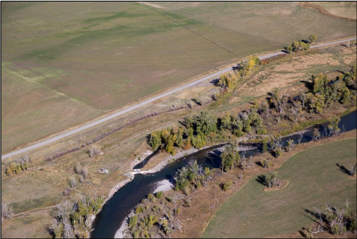
Figure 44. View downstream of diversion structure in area of minimal channel migration, RM 43.2L, Reach GR08 (Kestrel).
