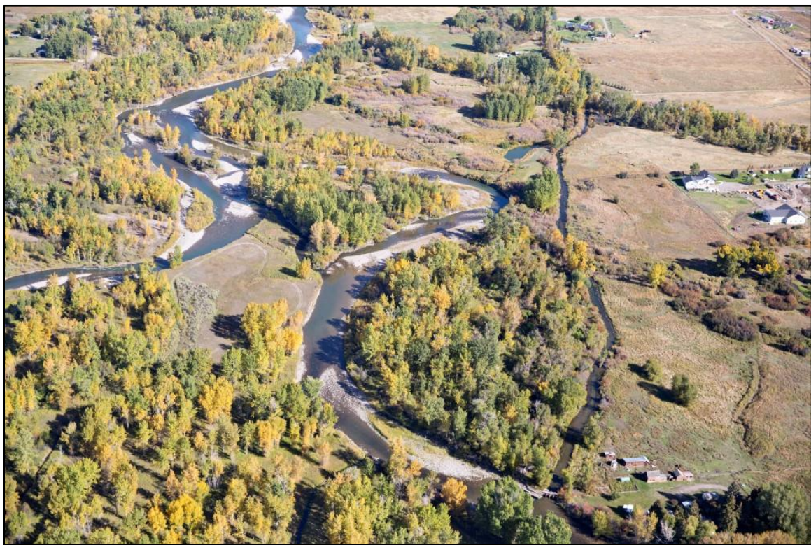
Figure 49. View downstream of Reach GR07 active meander migration towards a ditch at RM38.7R (Kestrel).
