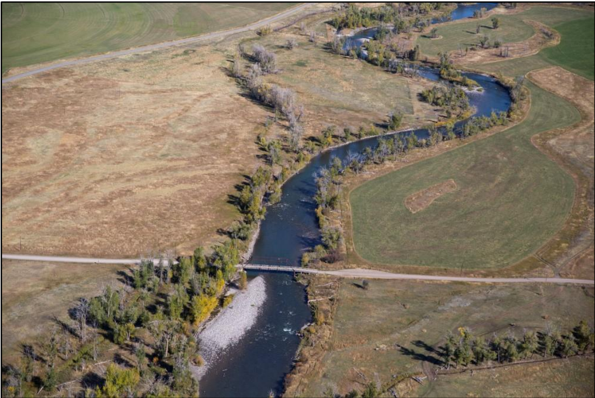
Figure 45. Increasing sediment storage and channel migration near West Williams Road Bridge, Reach GR08 (Kestrel).
