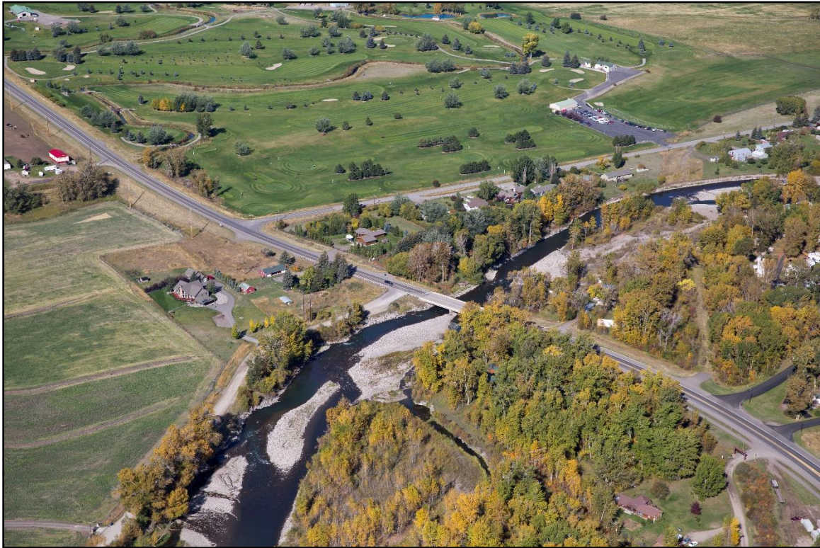
Figure 17. Extensive armor associated with the Norris Road bridge approach. (Kestrel)
