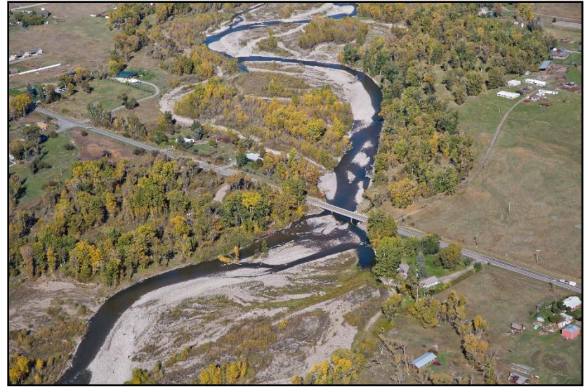
Figure 82. Amsterdam Road bridge on September 26, 2016. (Kestrel)
