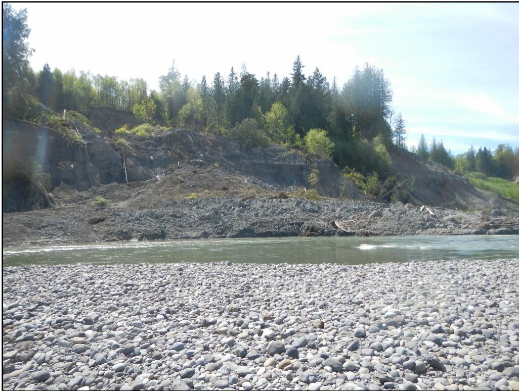
Figure 9. Hillslope failure on Nooksack River near Bellingham Washington on February 21, 2014 (K. Boyd).
