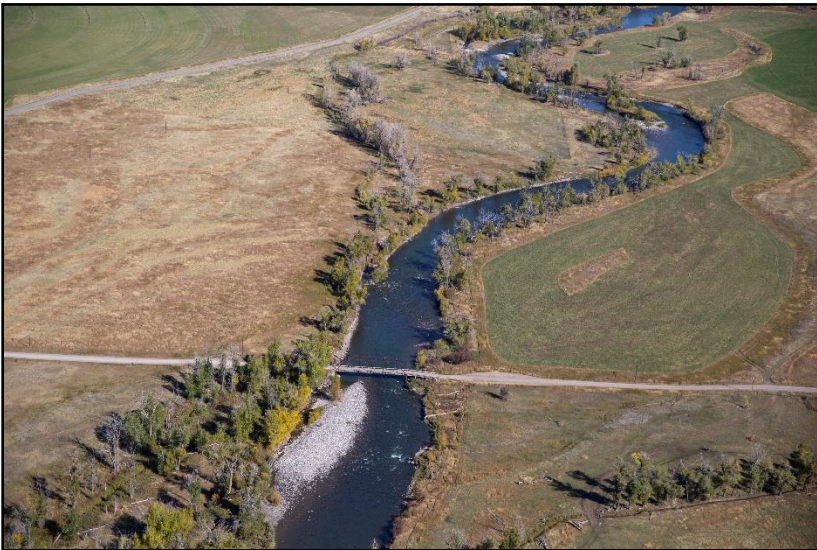
Figure 77. W Williams Road bridge on September 26, 2016. (Kestrel)
