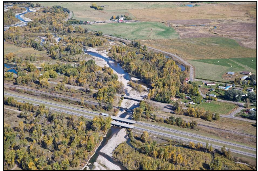
Figure 83. Bridge complex at I-90 on September 26, 2016. (Kestrel)
