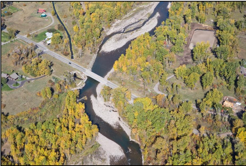
Figure 81. W Cameron Road bridge on September 26, 2016. (Kestrel)
