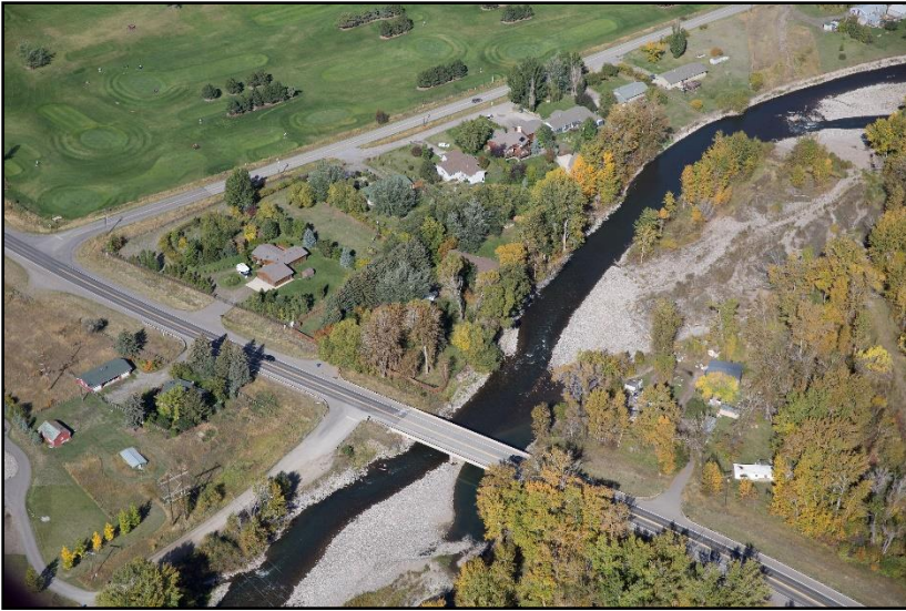
Figure 80. Norris Road bridge on September 26, 2016. (Kestrel)
