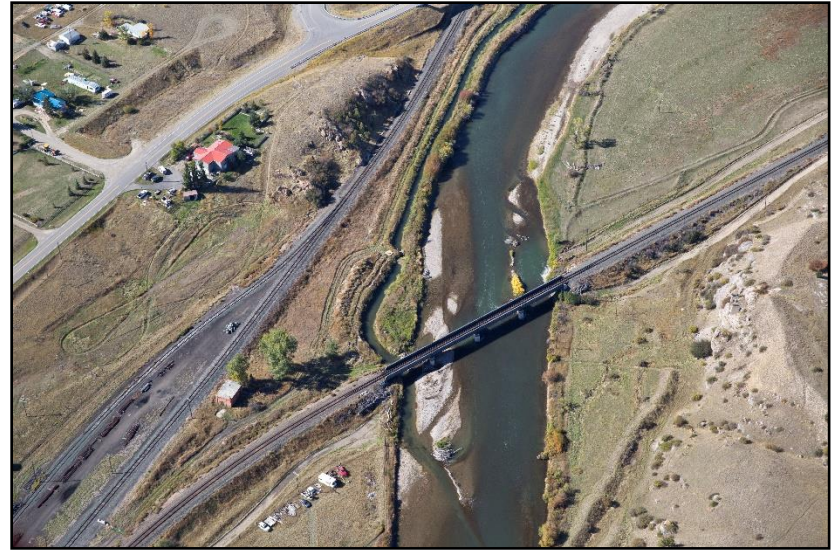
Figure 86. Railroad bridge at Logan on September 26, 2016. (Kestrel)
