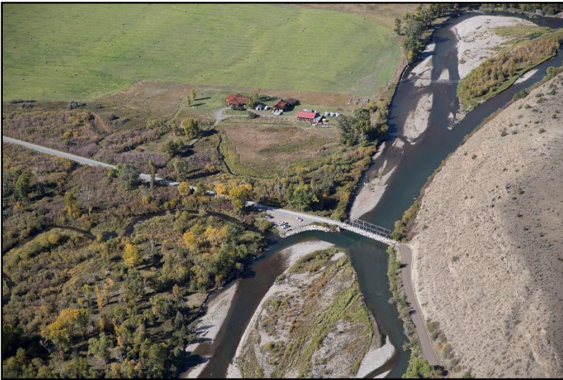
Figure 85. Nixon Gulch Road bridge on September 26, 2016. (Kestrel)
