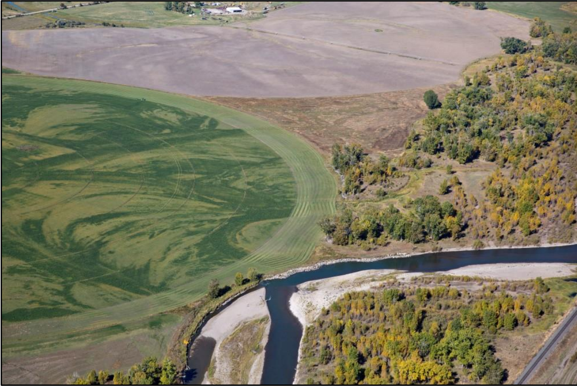
Figure 72. View downstream showing stream corridor narrowing between armored pivot field (left) and rail line (right) (Kestrel).
