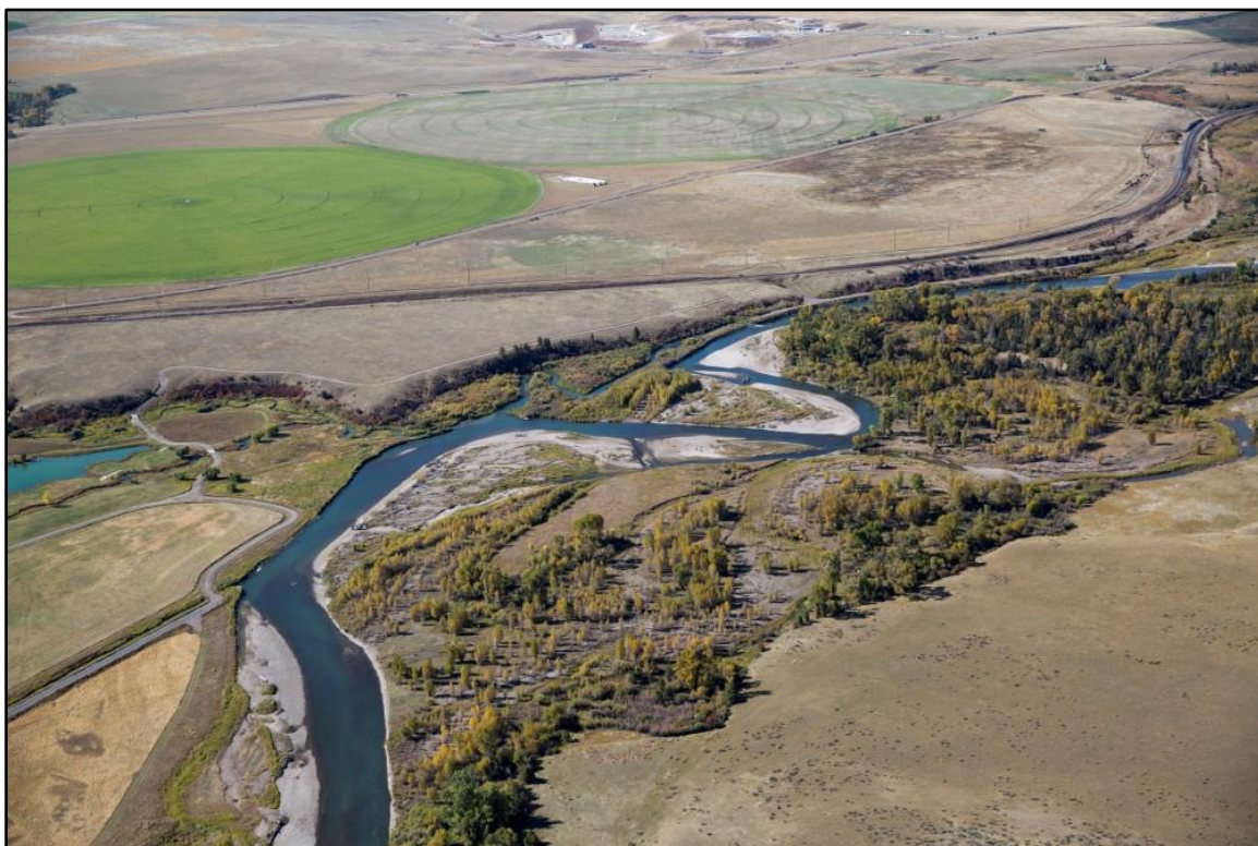
Figure 68. View downstream breached railroad grade and relocated road, Reach GR02 (Kestrel).
