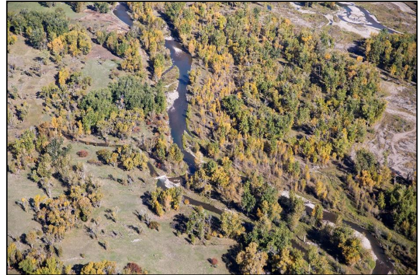
Figure 90. Diversion at RM 25.6, September 26, 2016 (Kestrel).
