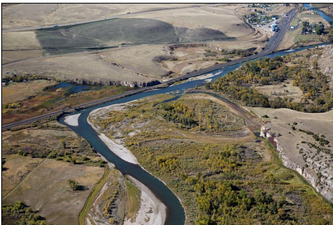
Figure 70. View downstream showing avulsion site and rail line isolation of historic floodplain, Reach GRO2 (Kestrel).
