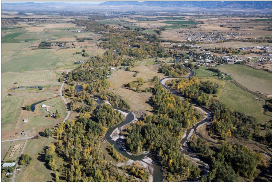
Figure 47. View downstream of Reach GR07 showing split flow approach to Gateway South Road bridge crossings (Kestrel).
