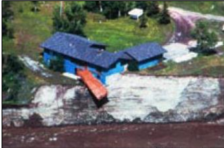
Figure 4. Yellowstone River home on high glacial terrace that was burned down in 1997 to prevent its undermining by the river.
