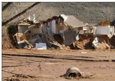
Figure 5. Photos from a 2005 in Saint George Utah, where homes several feet above the mapped floodplain were destroyed by channel migration ( www.Utahfloodrelief.com ).
