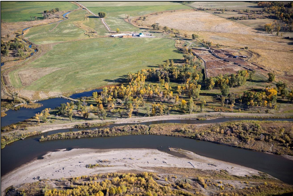
Figure 15. A 0.8-mile levee on the Lower Jefferson River. (Kestrel)
