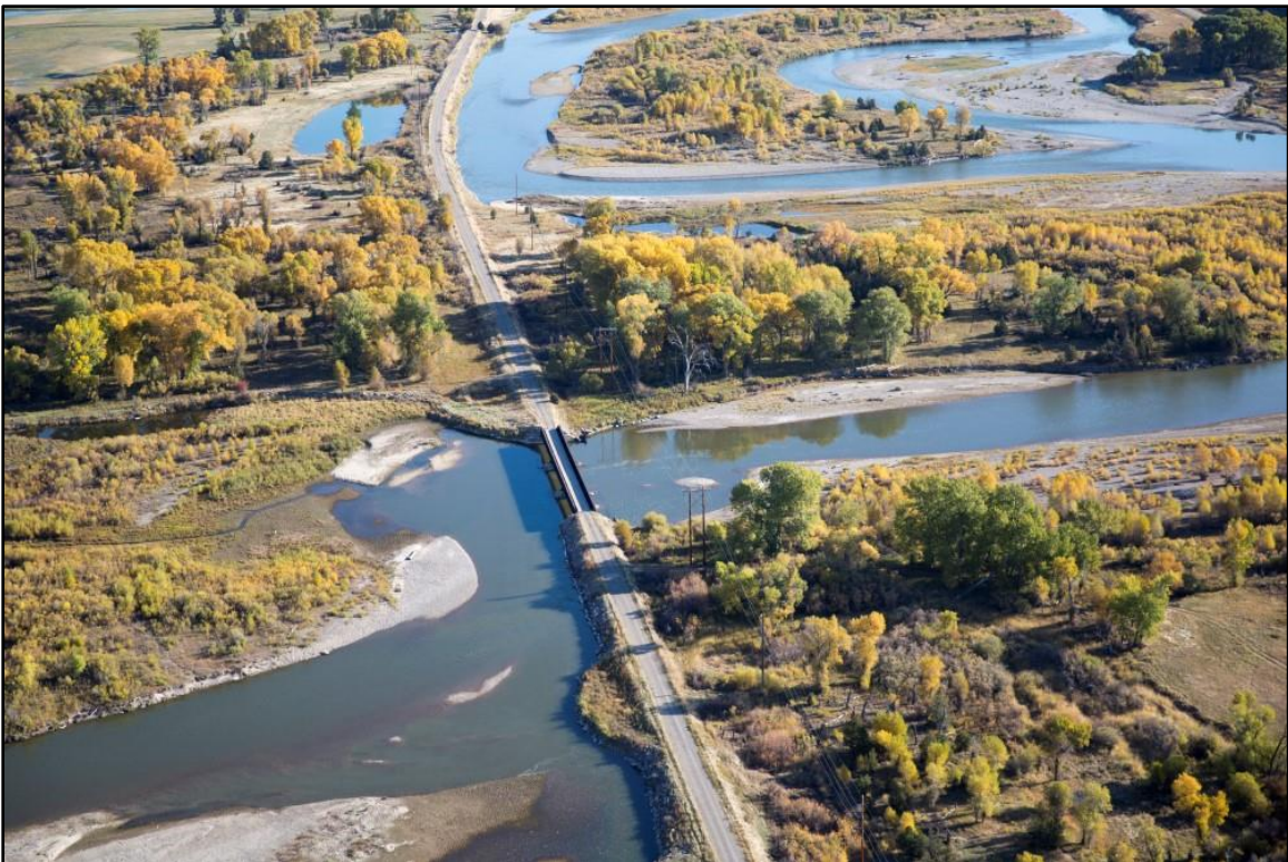
Figure 77. View down valley showing rail grade orientation to river corridor; Madison River is to right. (Kestrel)
