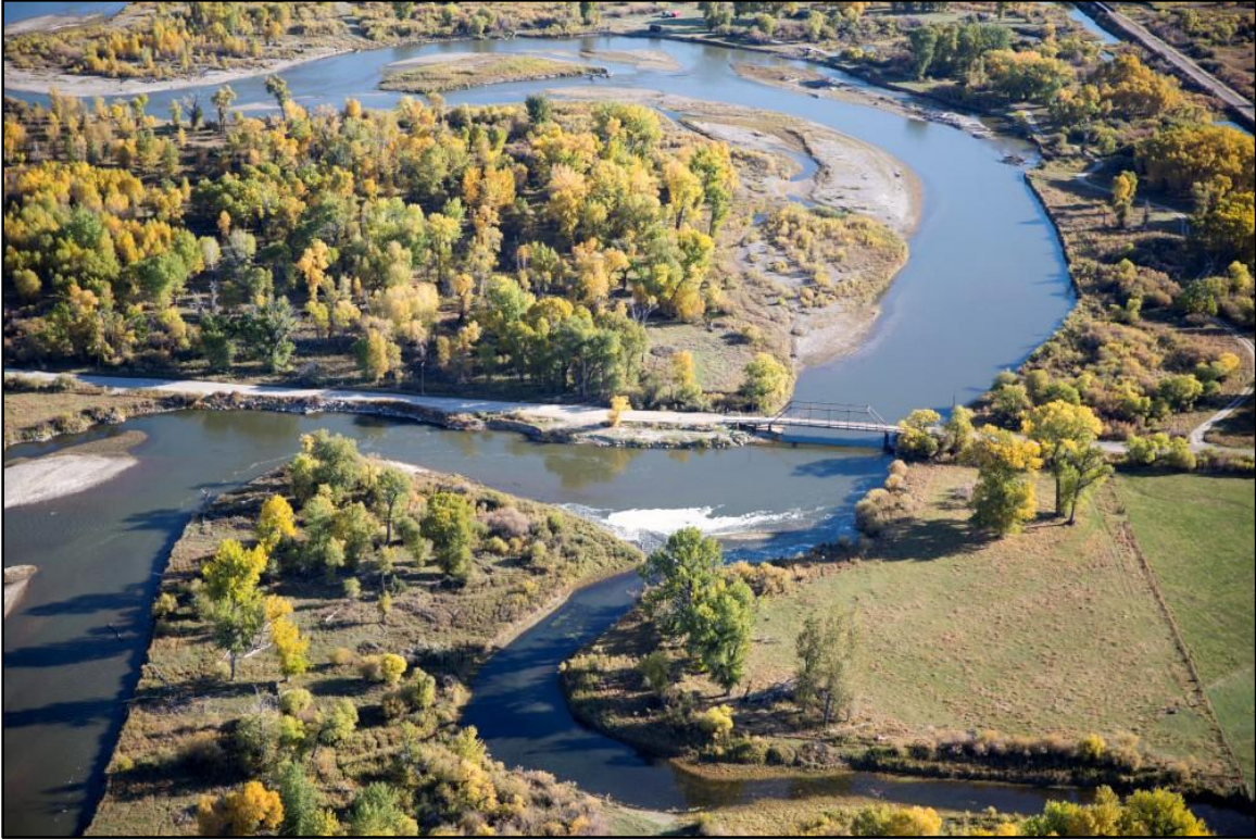
Figure 76. View downstream showing poor river alignment and bank armoring at Old Town Road Bridge over Jefferson River. (Kestrel)
