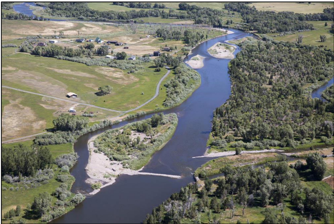
Figure 47. In-channel berming and side work at head of Parrot Canal, RM 68.54. (Kestrel)
