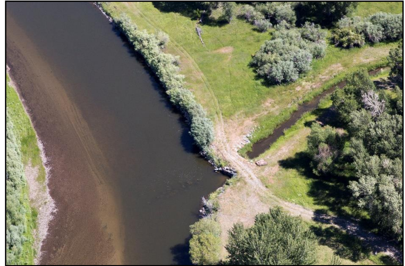
Figure 94. Diversion at RM 61.6, July 12, 2016 (Kestrel).
