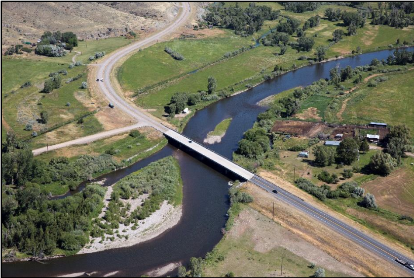
Figure 78. Iron Rod Bridge on July 12, 2016. (Kestrel)
