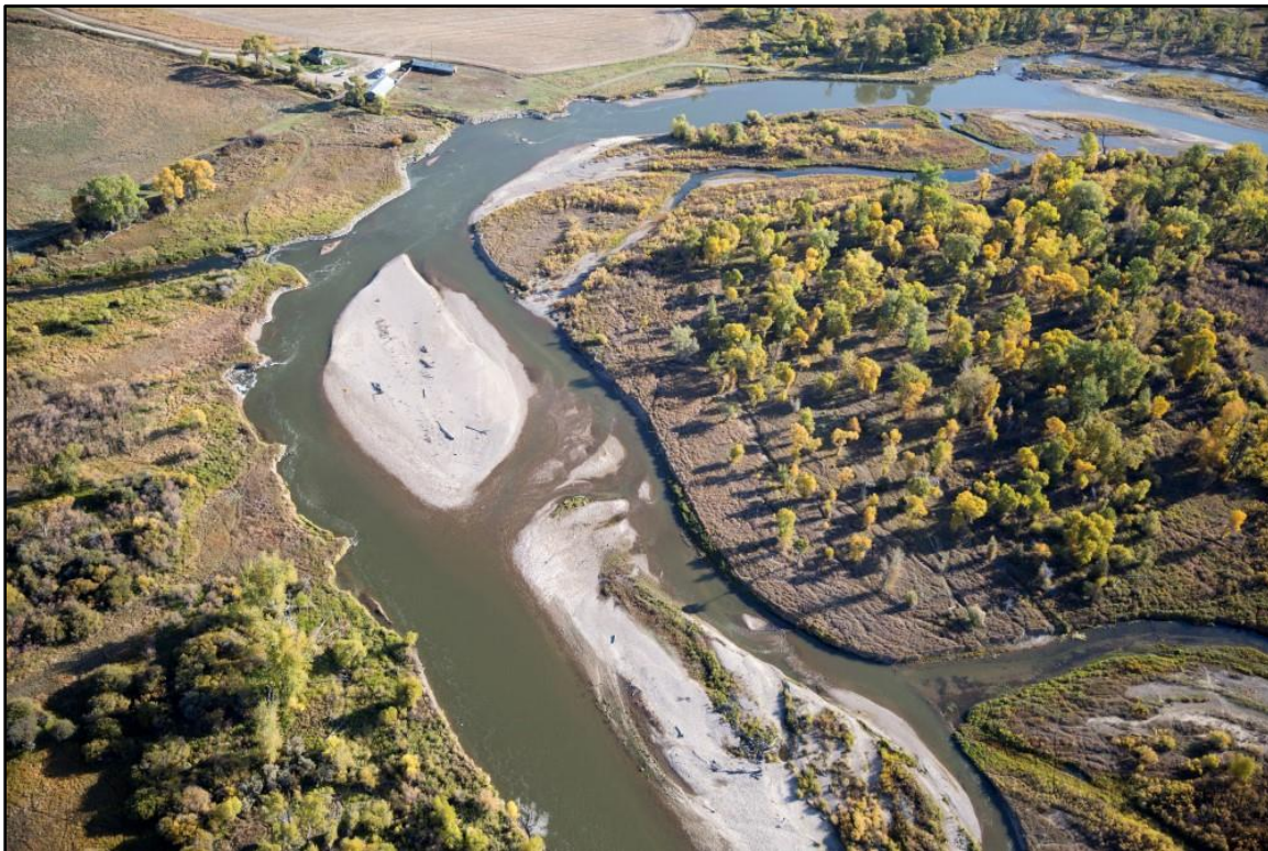
Figure 65. View downstream Reach JR04 showing left bank barbs with erosion between structures. (Kestrel)
