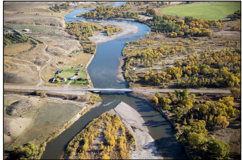
Figure 89. Hwy 2 bridge (Three Forks Frontage Road) on Sept. 30, 2016. (Kestrel)
