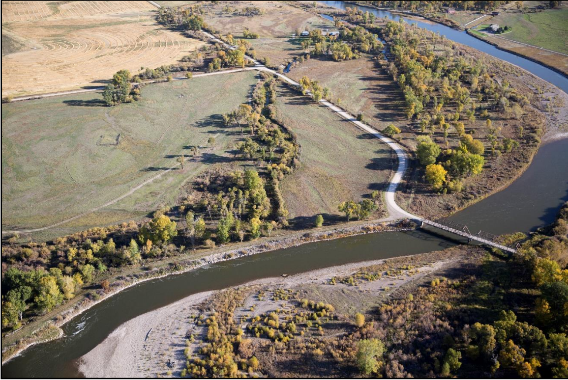
Figure 16. View (looking downstream) of the Meridian Bridge approach near Willow Creek showing a left bank levee. (Kestrel)
