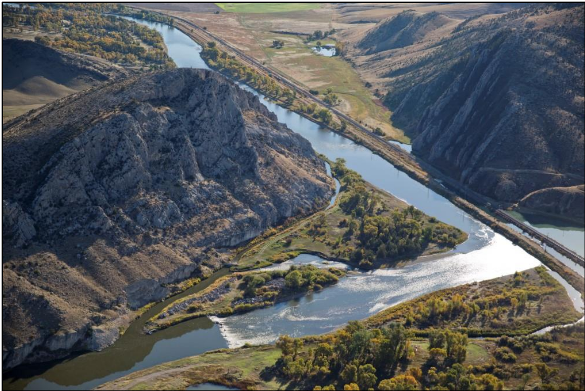
Figure 64. View downstream Reach JR05 showing Old Hale Diversion and floodplain encroachment by rail line. (Kestrel)
