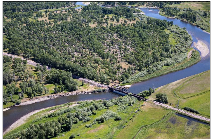
Figure 81. Railroad bridge downstream of Waterloo Road on July 12, 2016. (Kestrel)
