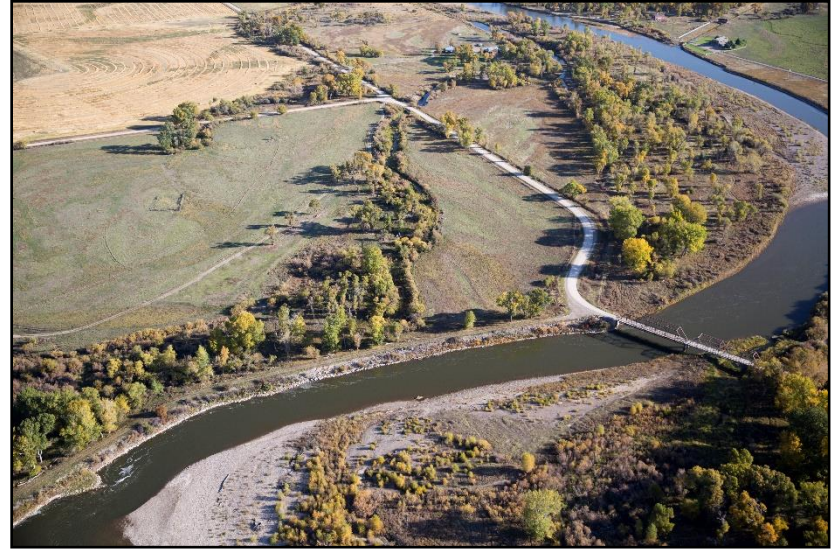
Figure 88. Meridian Road bridge on Sept. 30, 2016. (Kestrel)
