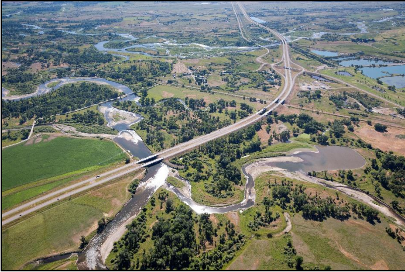
Figure 90. Bridge grouping at Three Forks (I-90, Old Town Road) on July 21, 2016. (Kestrel)
