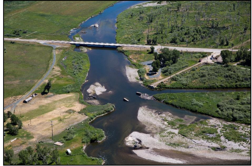
Figure 84. Cardwell Bridge on July 12, 2016. (Kestrel)
