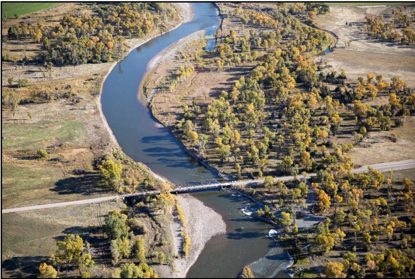
Figure 87. Williams Road bridge on Sept. 30, 2016. (Kestrel)
