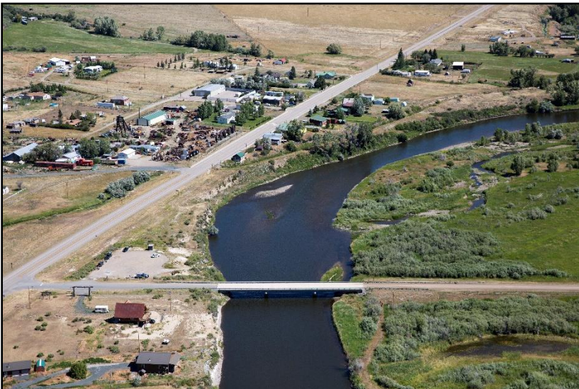
Figure 79. Primrose Lane Bridge on July 12, 2016. (Kestrel)
