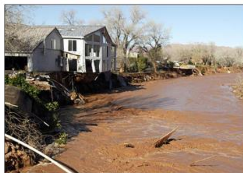
Figure 5. Photos from a 2005 in Saint George Utah, where homes several feet above the mapped floodplain were destroyed by channel migration ( www.Utahfloodrelief.com ).
