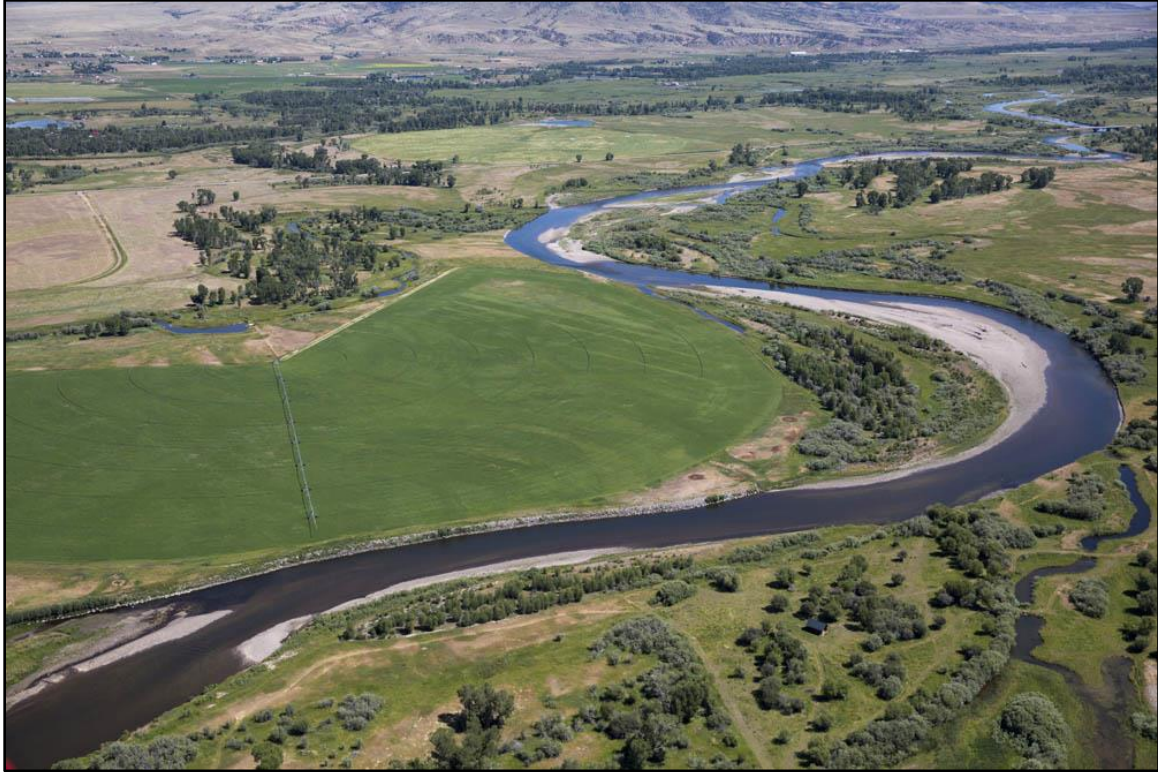
Figure 57. View downstream of Reach JR08 showing meander core irrigation and left bank armor. (Kestrel)
