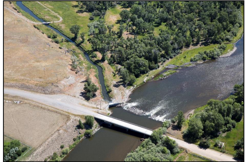
Figure 80. Waterloo Road bridge on July 12, 2016. (Kestrel)
