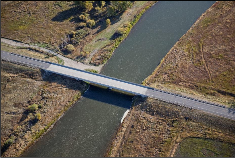
Figure 86. Sappington Bridge on Sept. 30, 2016. (Kestrel)
