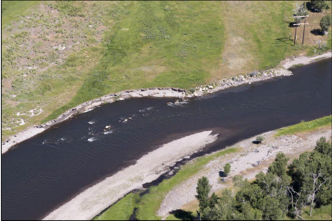
Figure 44. Flanked left bank riprap in channel, RM 71.8L. (Kestrel)
