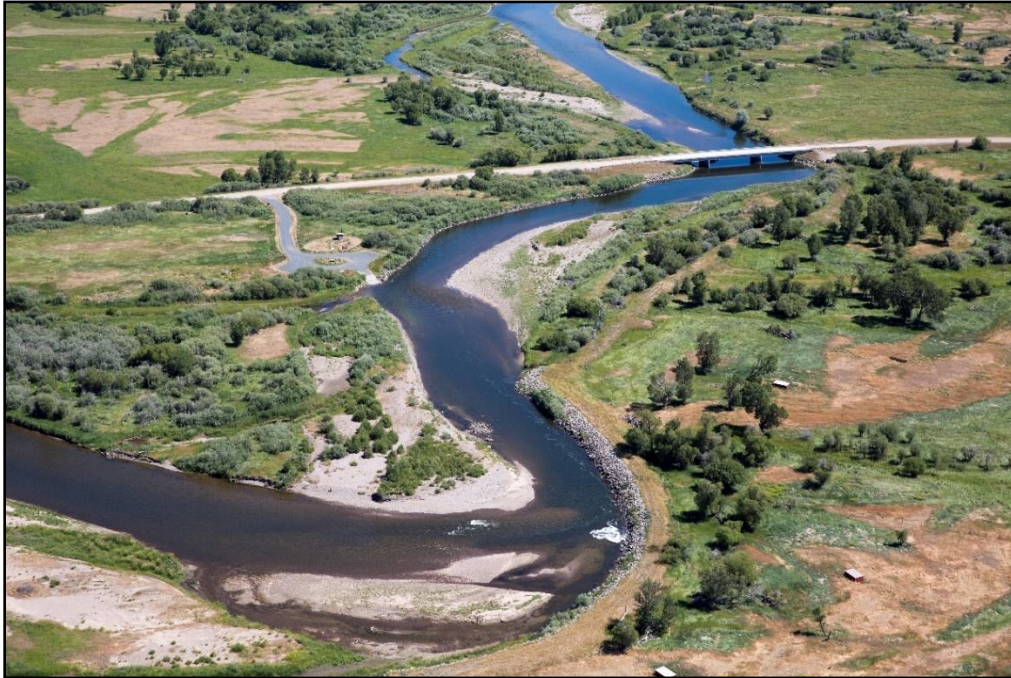
Figure 17. Extensive armor associated with the Kountz Road bridge approach. (Kestrel)
