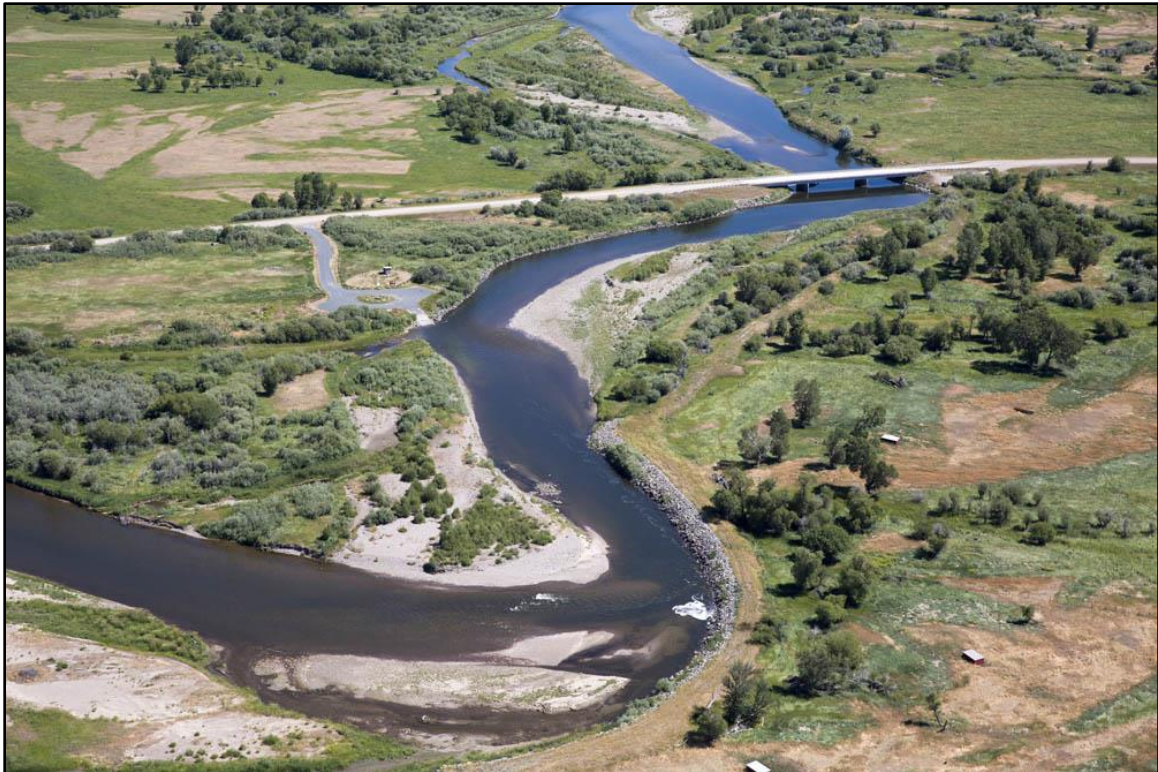
Figure 58. View downstream of Kountz Road Bridge showing dense armor on approach. (Kestrel)
