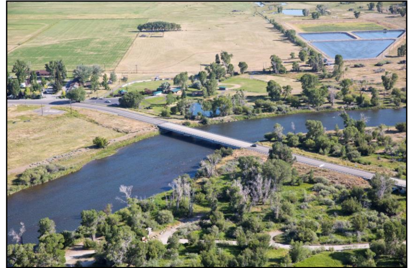
Figure 69. Highway 287 Bridge on July 21, 2016. (Kestrel)
