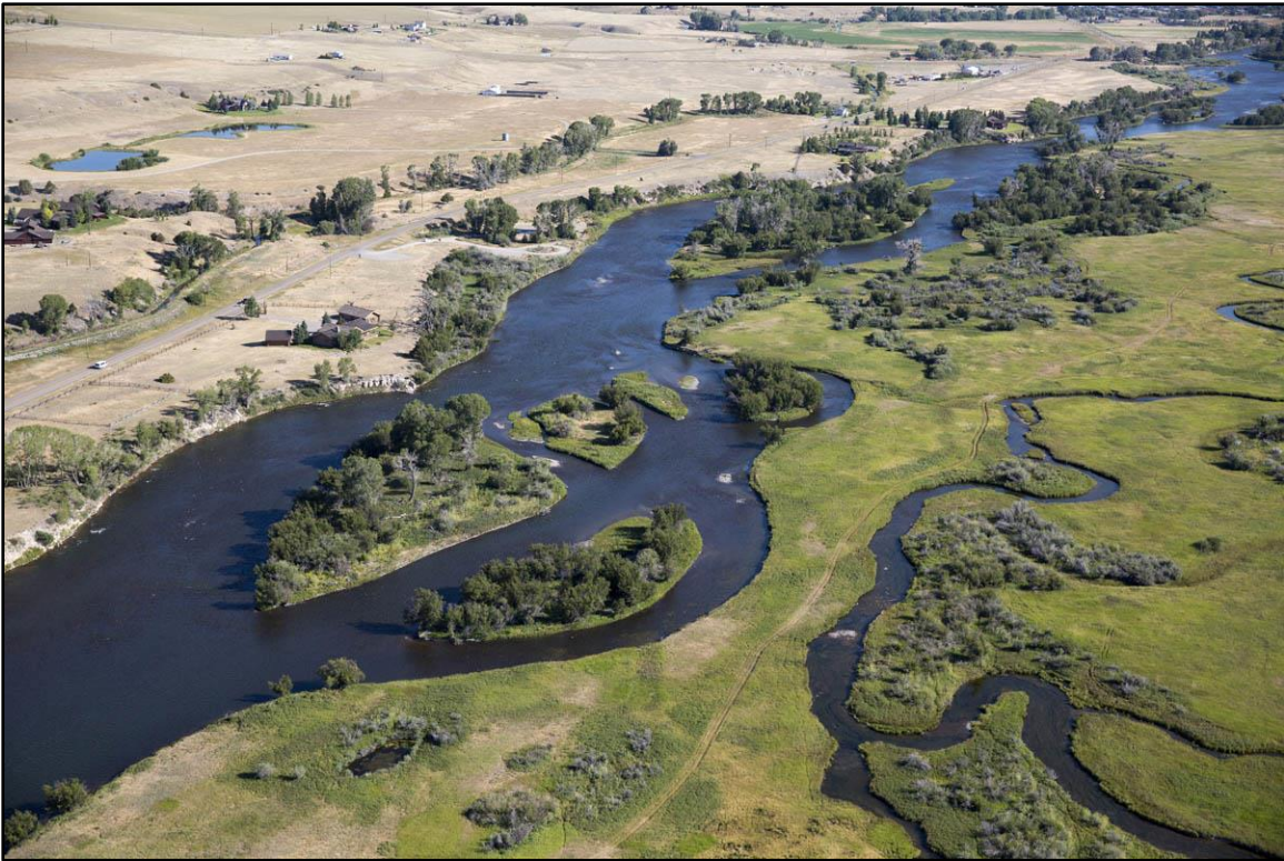
Figure 46. View downstream showing avulsion risk into spring creek, RM 53.9. (Kestrel)
