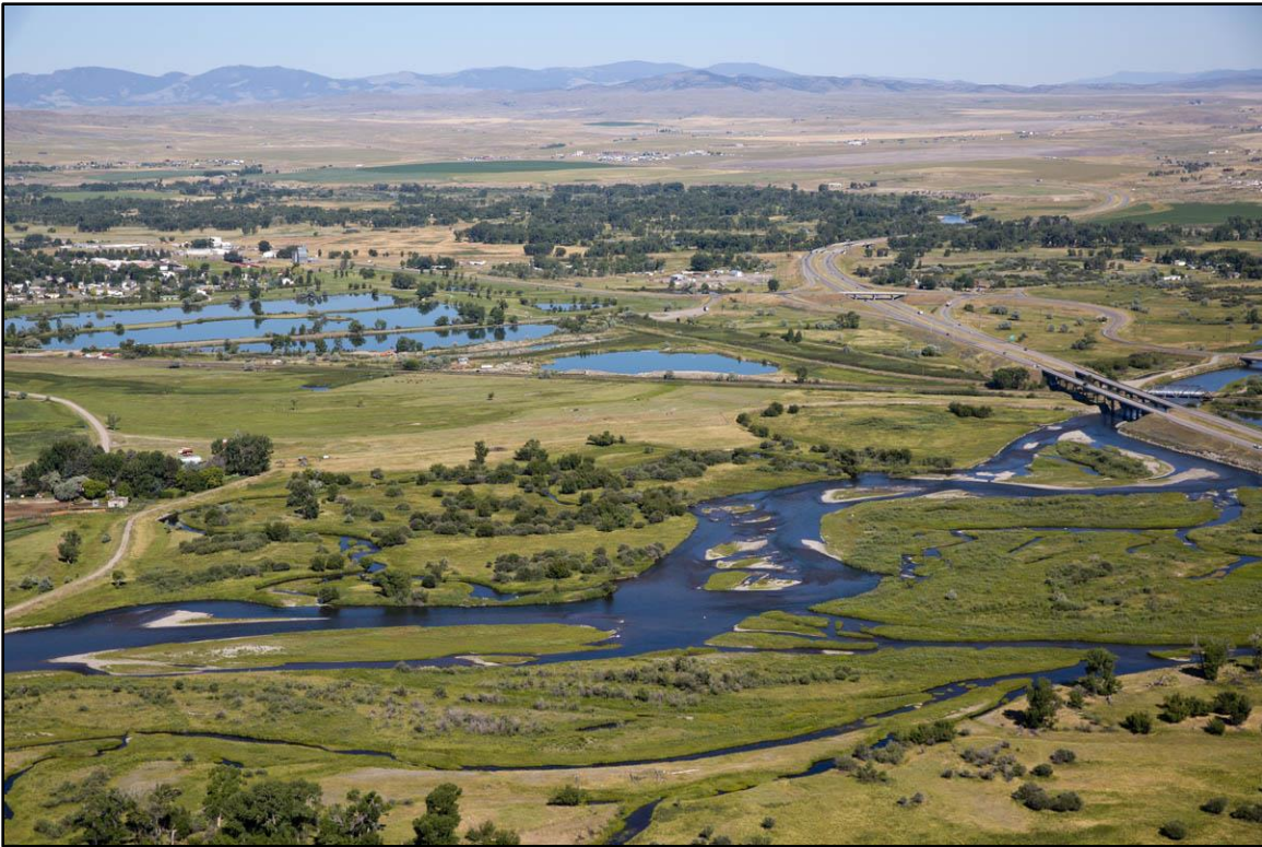
Figure 64. View downstream showing corridor constriction at I-90 bridge on right. (Kestrel)
