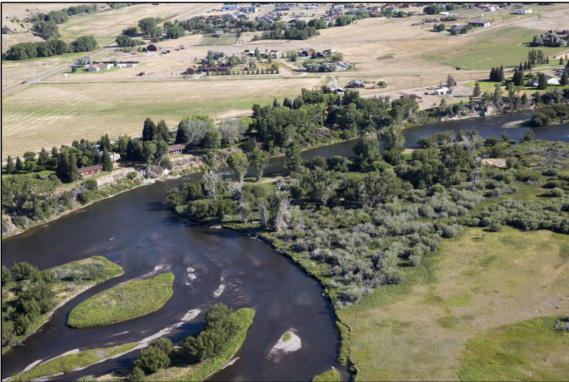
Figure 47. View downstream showing development along bluff line on the outskirts of Ennis. (Kestrel)
