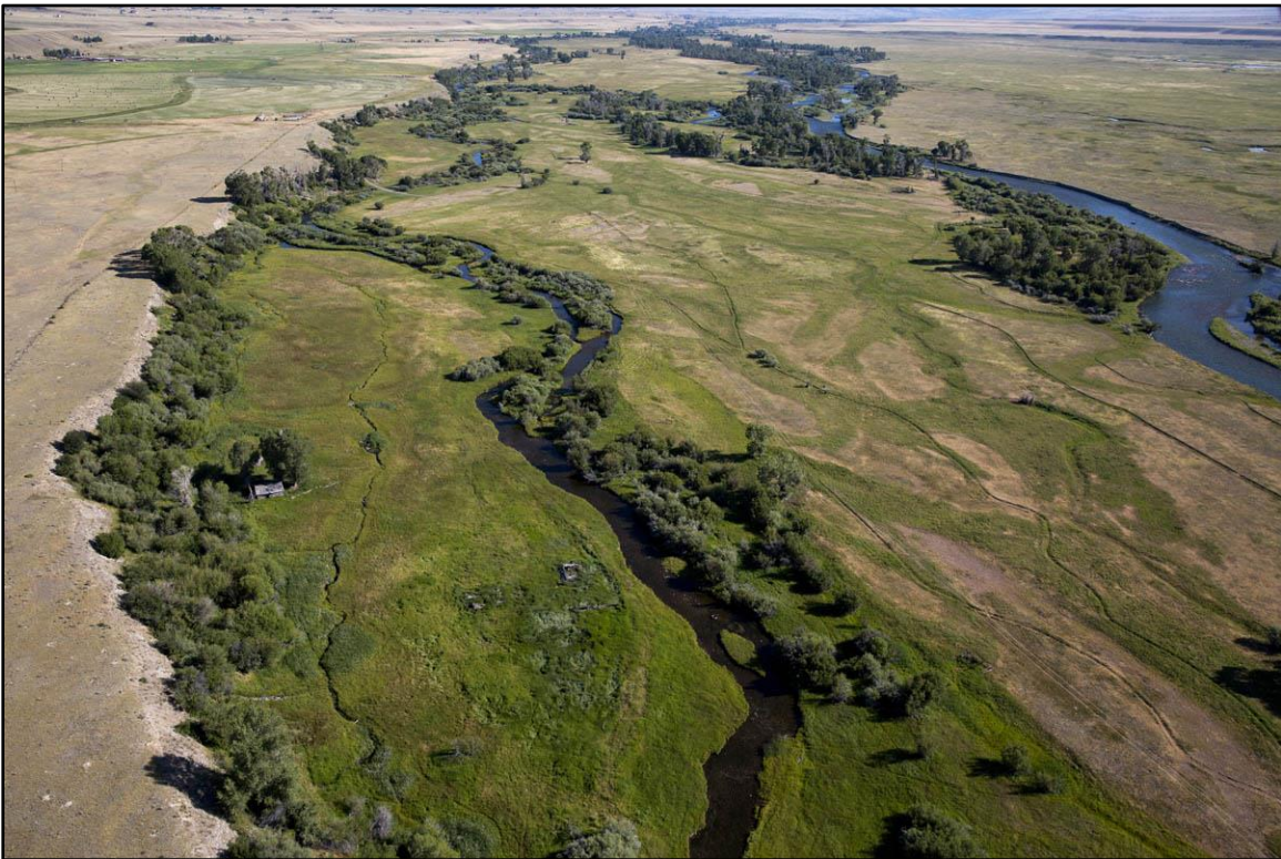
Figure 42. View downstream from near Varney Bridge showing Blaine Spring Creek avulsion risk area; main channel is to right. (Kestrel)
