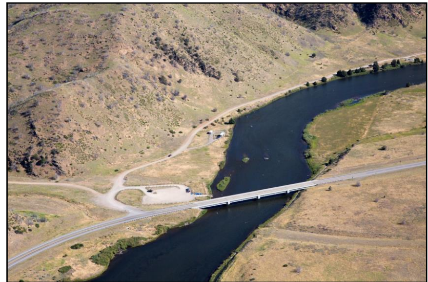
Figure 71. Norris Road (Highway 84) bridge on July 21, 2016. (Kestrel)
