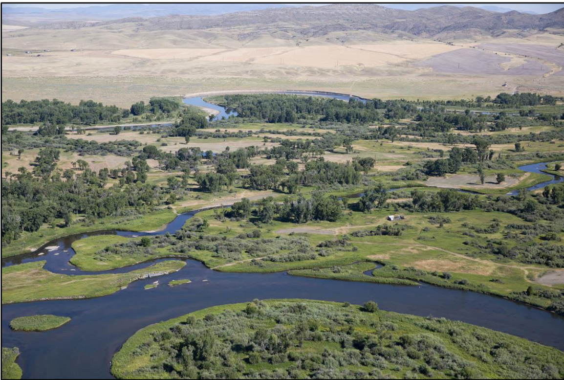
Figure 66. Lower Madison (foreground) showing breached dike. (Kestrel)
