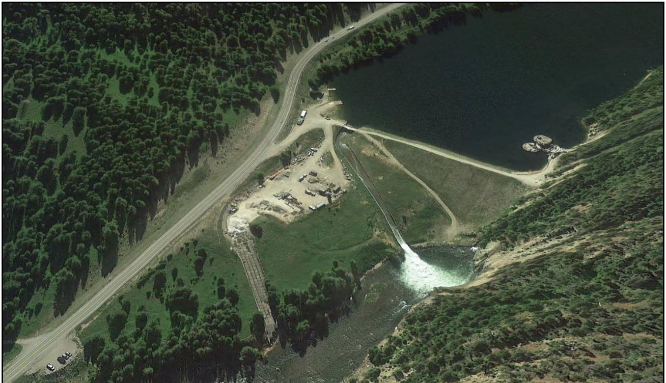
Figure 13. Hebgen Dam, Montana. (Google Earth).
