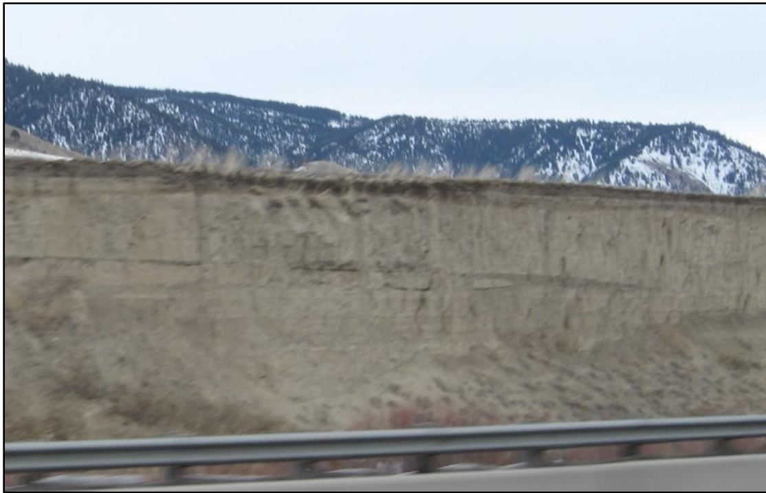
Figure 14. Fine-grained glacial Lake Missoula deposits forming Clark Fork River bankline as seen from I-90.
