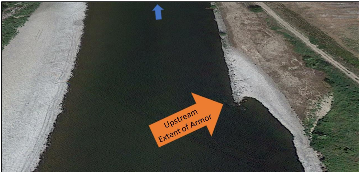
Figure 117. Google Earth image showing scour behind armor at RM 197.
