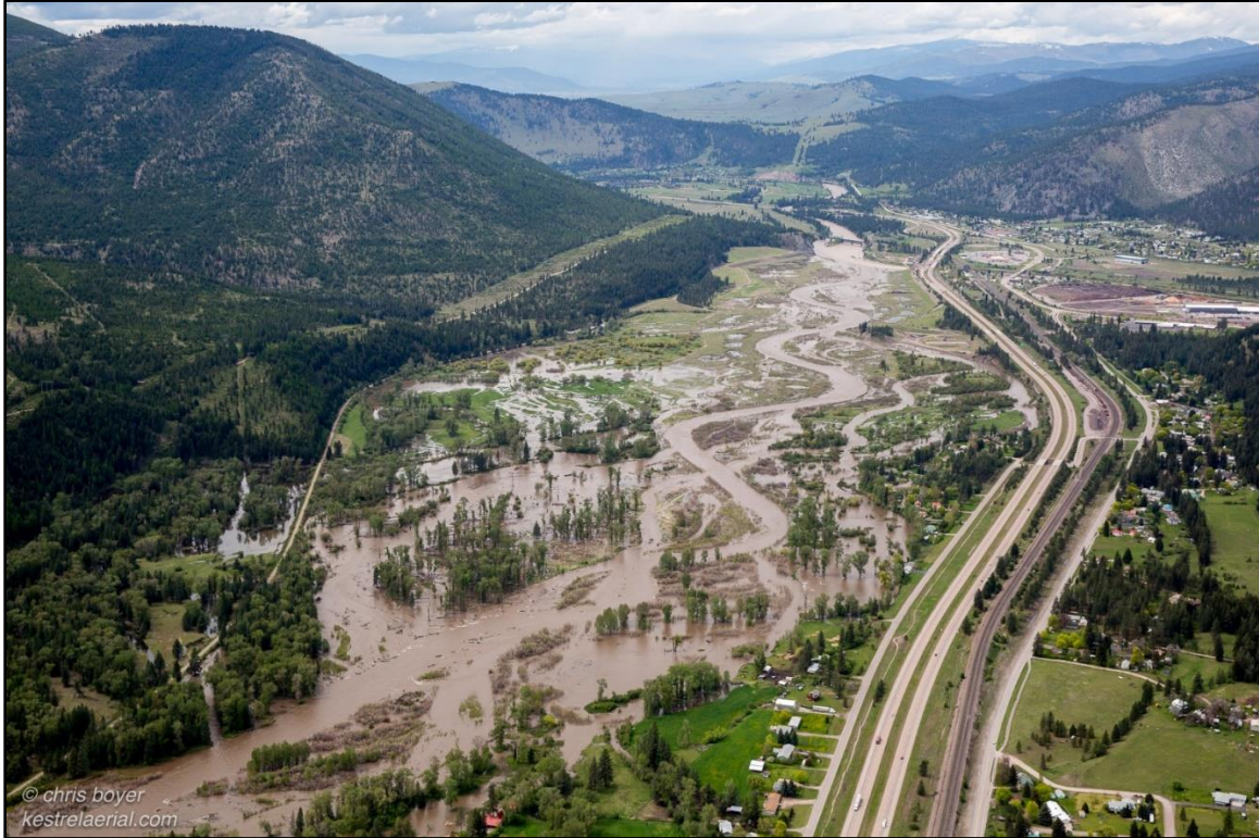
Figure 60. View downstream through Milltown Dam restoration area showing constructed channel, wetland features, and broad inundation during the 2018 flood event. Connelly Loop feeds the cluster of homes in center-right of photo (May 10, 2018).
