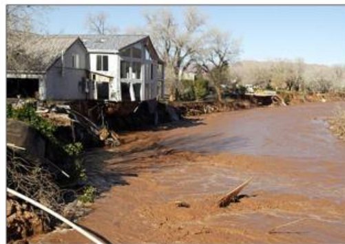
Figure 6. Photos from a 2005 flood event in Saint George Utah, where homes several feet above the mapped floodplain were destroyed by channel migration ( www.Utahfloodrelief.com ).
