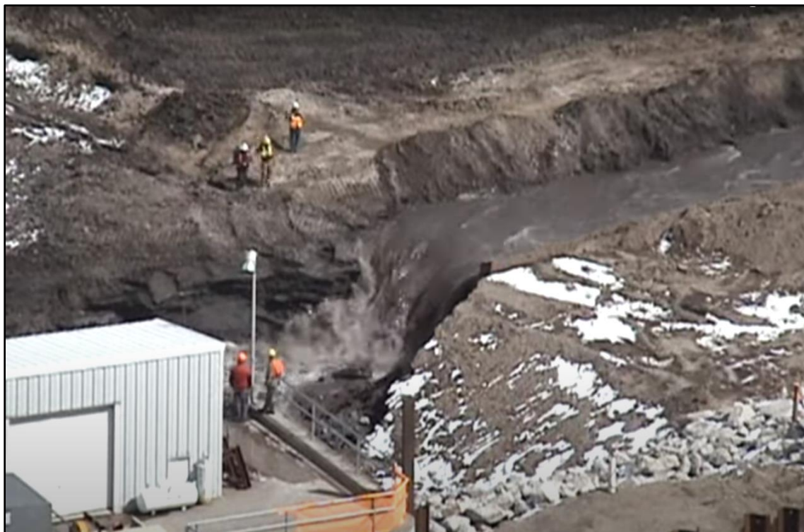
Figure 106. Large headcut formed as Milltown Dam was breached on March 28, 2008 showing base level lowering that drove channel downcutting upstream and accelerated sediment delivery below (extracted from a youtube video by American Whitewater).
