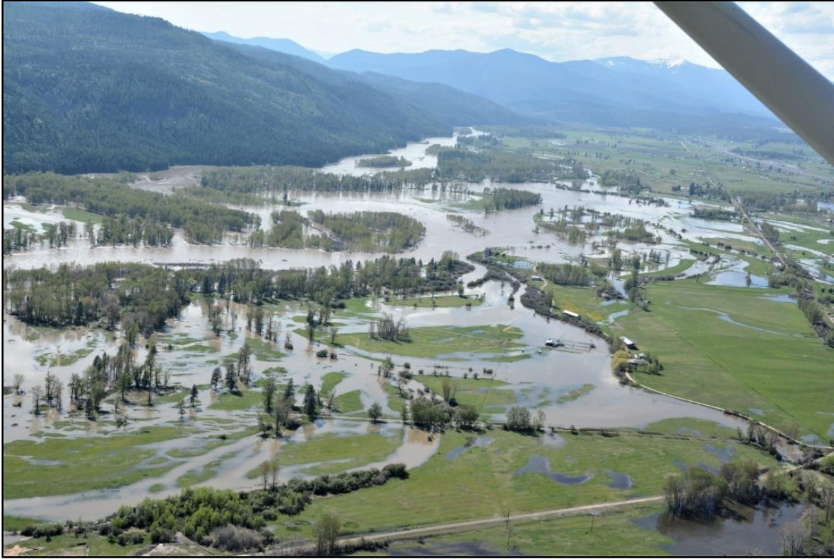
Figure 90. View downstream of the upper portion of Reach CF10 showing floodwaters accessing floodplain swales (CAP May 8, 2018).
