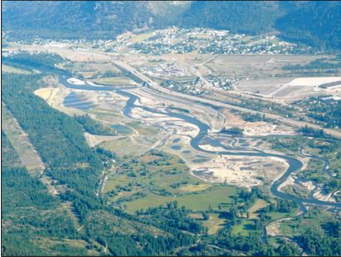
Figure 105. View downstream showing Milltown Dam Removal and Restoration Site shortly after project completion (River Design Group)
