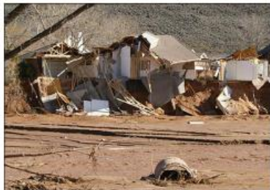
Figure 6. Photos from a 2005 flood event in Saint George Utah, where homes several feet above the mapped floodplain were destroyed by channel migration ( www.Utahfloodrelief.com ).
