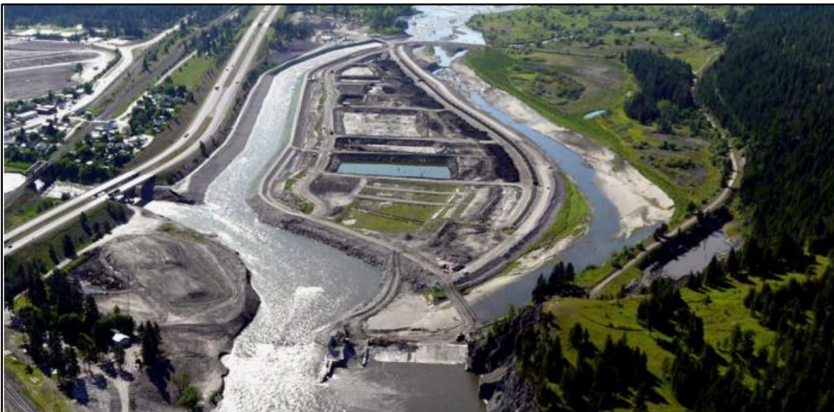
Aerial view of remediation and restoration activities at the site, 2009.
