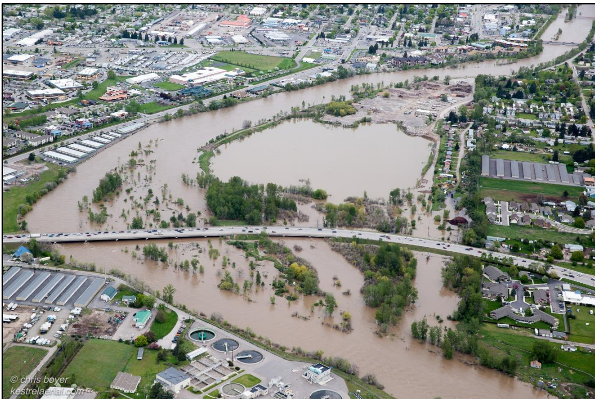
Figure 66. View upstream of Reserve St Bridge showing gravel pit and high flow paths under bridge to the right of the main channel (May 10, 2018).
