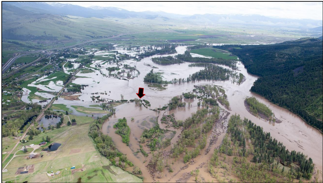
Figure 93. View upstream at RM 192 showing high risk avulsion route (red arrow) (CAP May 8, 2018).
