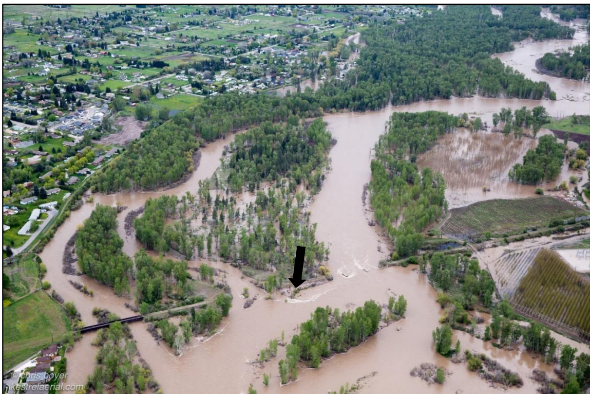
Figure 70. View downstream showing flow paths through abandoned rail line crossing; rock-reinforced utility pole is noted by black arrow (May 10, 2018).
