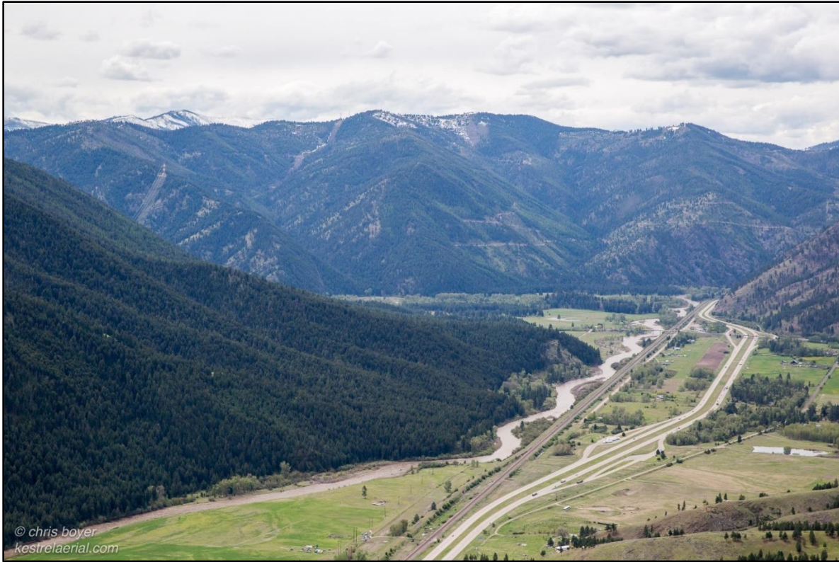
Figure 47. View west of Reach CF01 showing corridor confinement by valley wall and railroad—Rock Creek confluence is in background.
