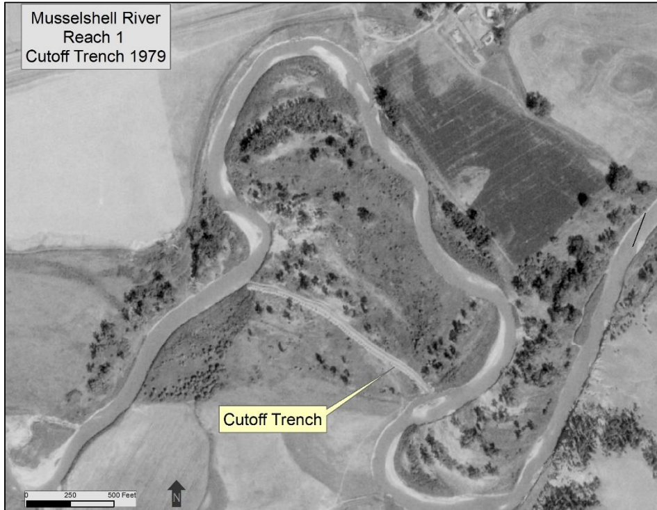
Figure 38. 1979 image showing newly excavated cutoff trench at RM 163.4.
