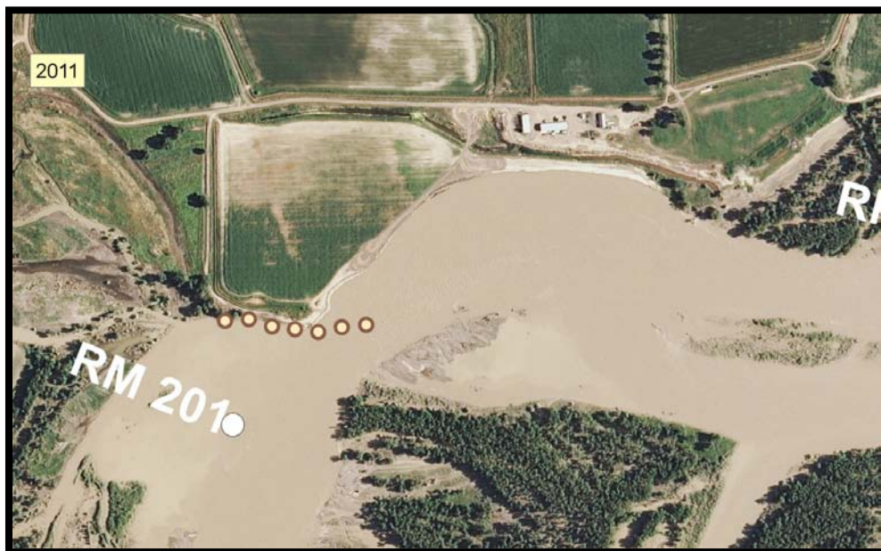
Figure 4. In June of 2011, high water eroded the bankline behind a section of rock riprap (brown dots) and migrated over 600 feet northward at this location on the Yellowstone River; nearly 700 feet of emergency riprap was placed to protect threatened buildings.
