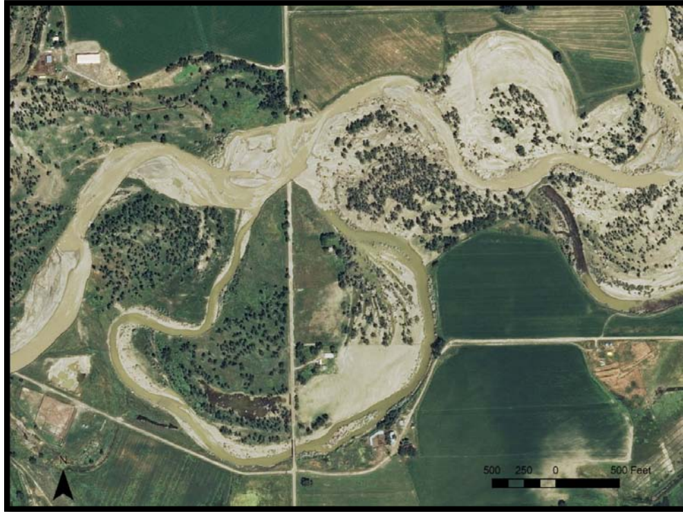
Figure 3. Avulsion at Harvey Bridge Road on the Musselshell River (flow is from left to right) requiring the construction of a new bridge.
