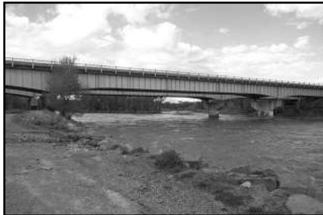
Photo 34. Interstate 90 Bridge in Livingston, 2002. Photo courtesy of M. Gilbert.
