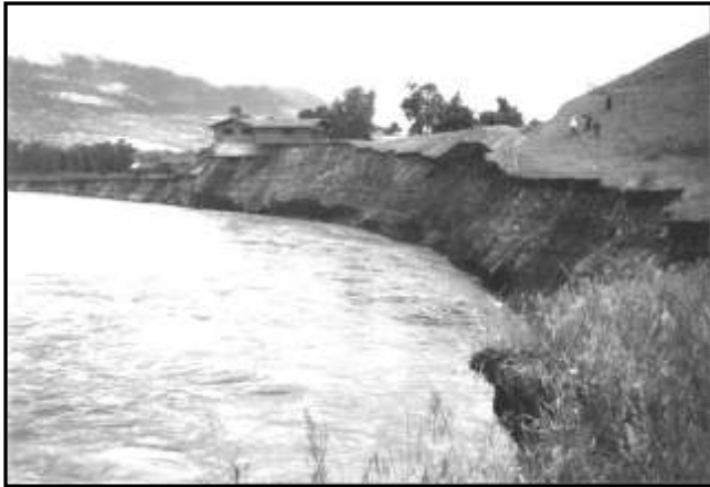
Photo 6. House lost in high water in 1997. Photo source unknown.
