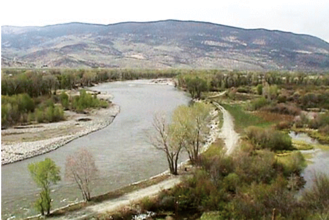
Bank stabilization using rip-rap along the Yellowstone River.
