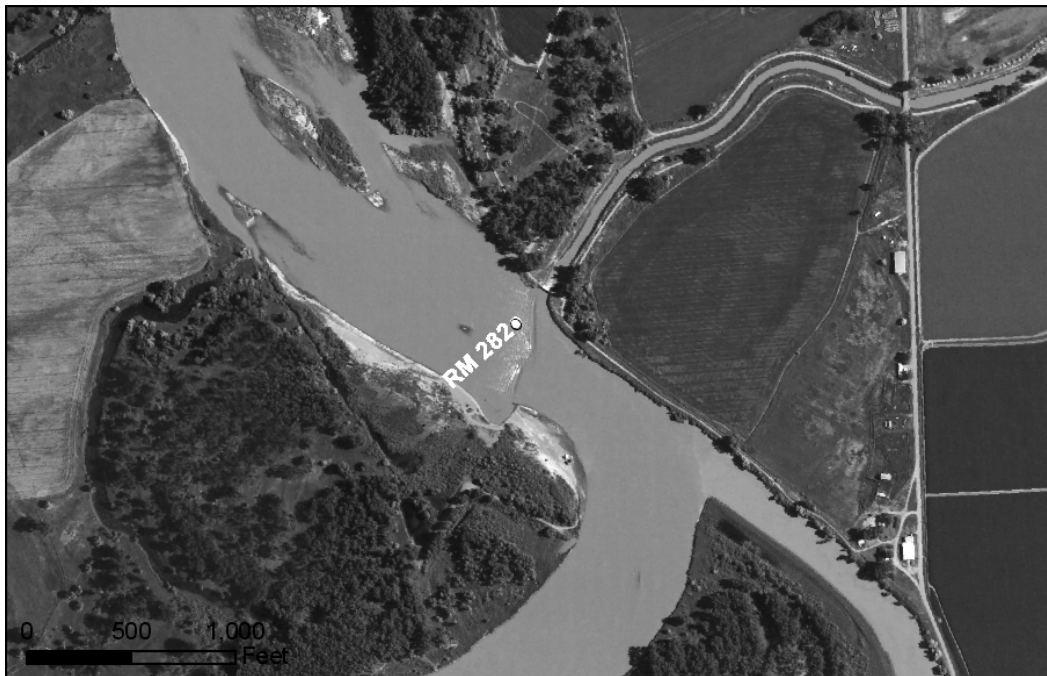
Plate 4. 2005 aerial image of Yellowstone Ditch Diversion Dam.
