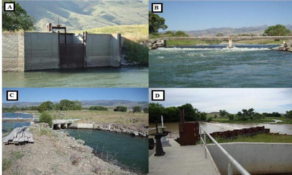
Figure 3.17 Examples of diversion types in the Yellowstone River Basin (A. Headgate without diversion; B. Side channel diversion; C. Multiple headgate partial channel diversion; D. Entire channel diversion with multiple headgates).
