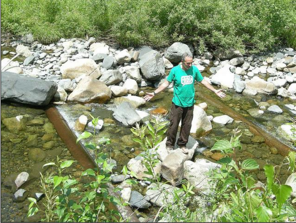
Figure 5. Exposure of two pipelines on small creek in Vermont. ( http://world.350.org )
