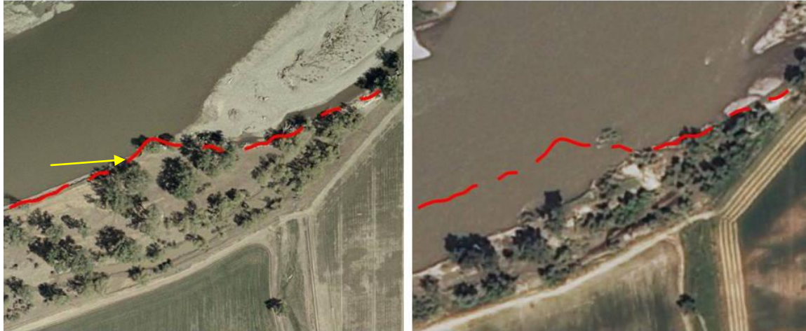
Figure 29. Site 14 bankline showing 2004 (left) and 2011 (right) conditions; red line is 2004 bankline and yellow is upstream end of armor in 2004. Pipeline runs parallel to field road on lower portion of image.
