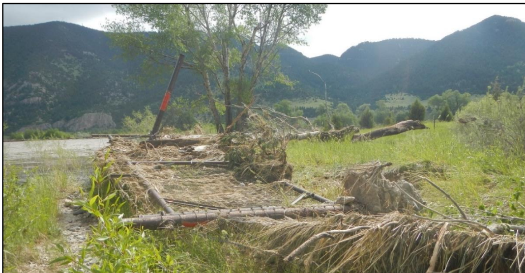
Figure 27. Miles of fencing were destroyed during the 2022 flood.
