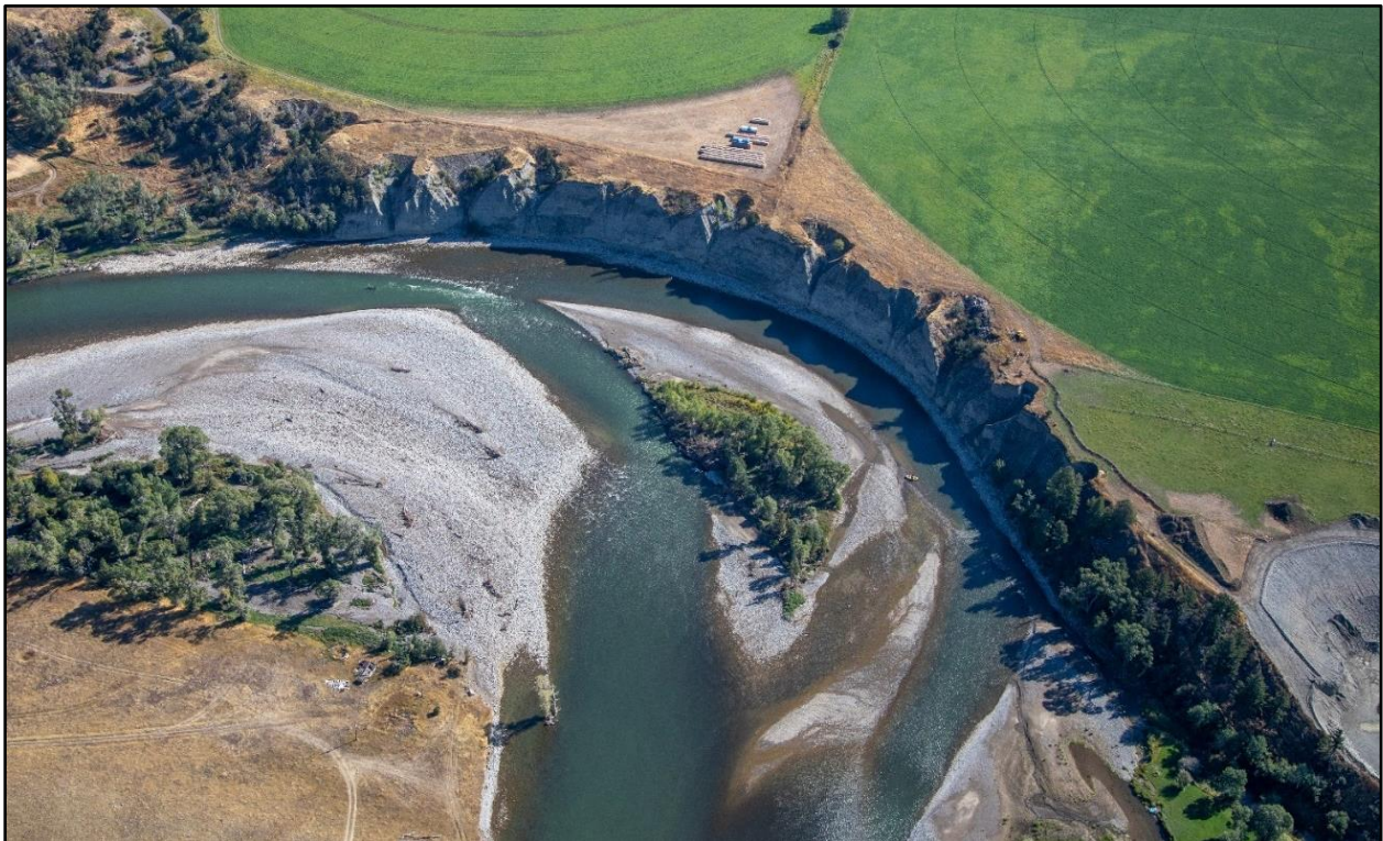
Figure 18. High eroding outwash terrace against river at the Weeping Wall below Pine Creek (Kestral Aerial Services),
