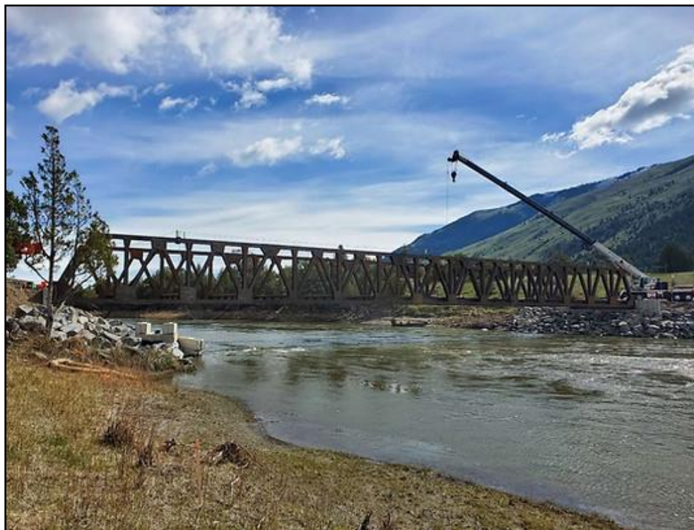
Figure 50. Reconstruction of the Carbella Bridge following the flood (Stahly Engineering).
