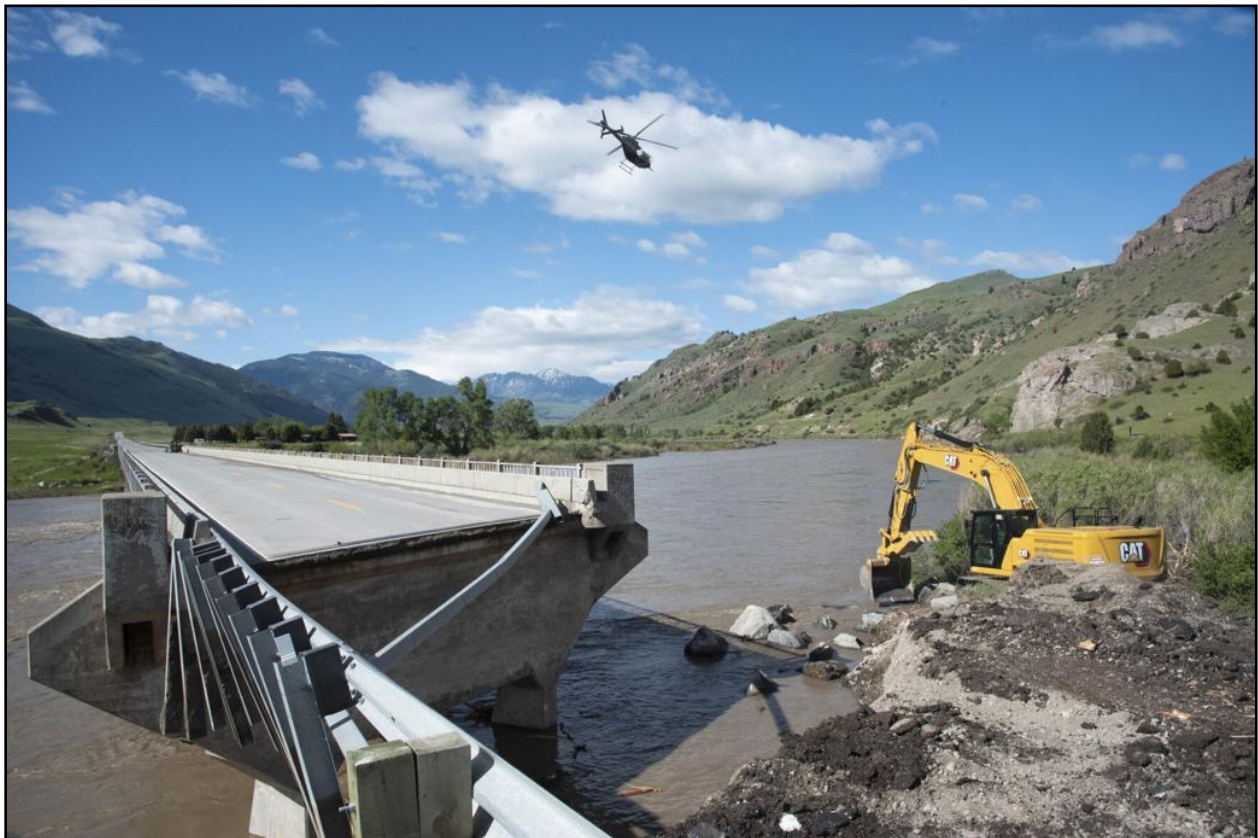
Figure 52. Point of Rocks Bridge showing where the northern approach was flanked during the flood. (Samuel Wilson/Chronicle/Report for America).
