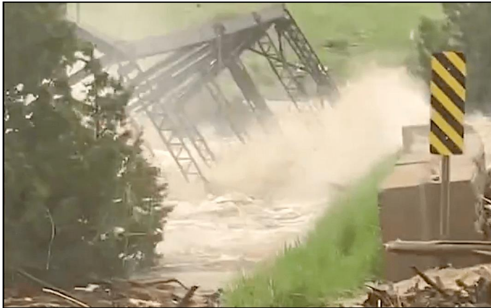
Figure 49. The Carbella Bridge seen as it collapsed into the river (source unknown).
