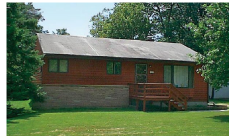
Elevated house on Crawl Space from FEMA 511, “Reducing Damage from Localized Flooding”. Photo credit: French & Associates
