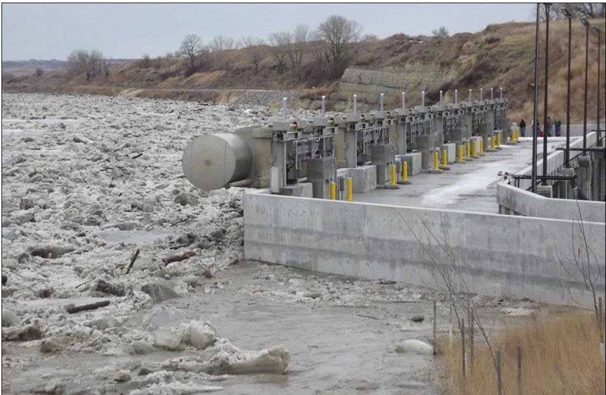
**Figure 4-18** Ice action at Intake Diversion Structure, 2014
