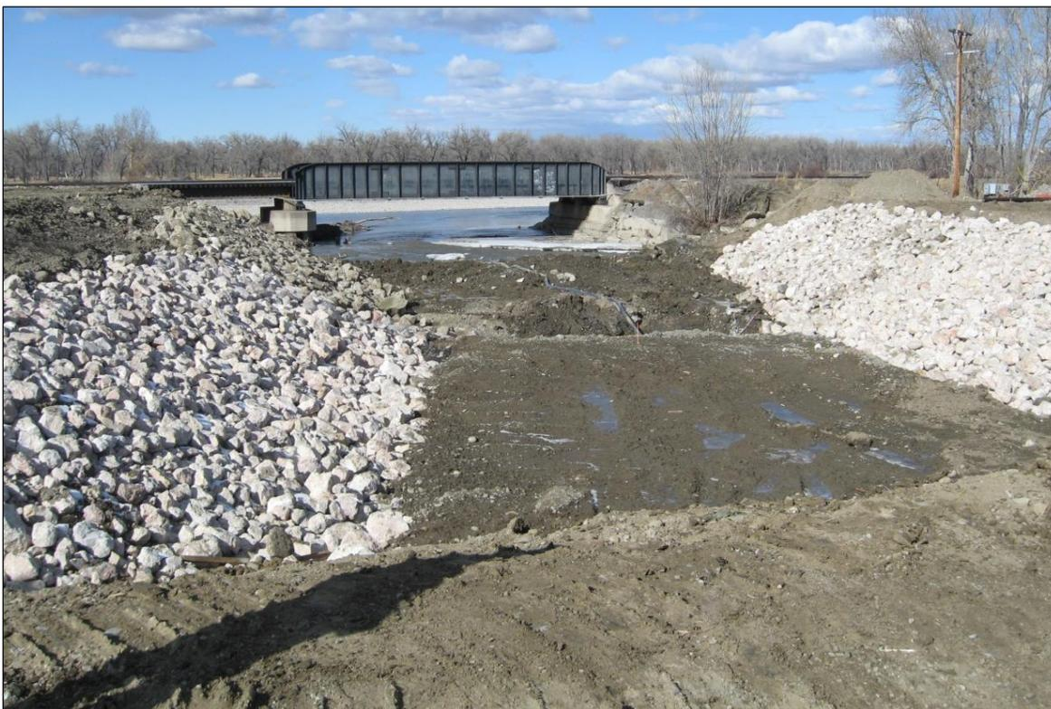
**Figure 4-23** View downstream of lower Pryor Creek towards Yellowstone River, showing creek passing over newly constructed Huntley Canal siphon, which passes under creek from left to right below riprapped banks
