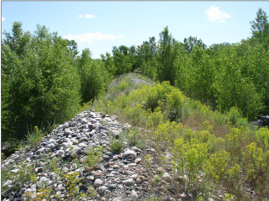
**Figure 8-1** Gravel dike on the floodplain near Billings, built to protect a residential development from flooding
