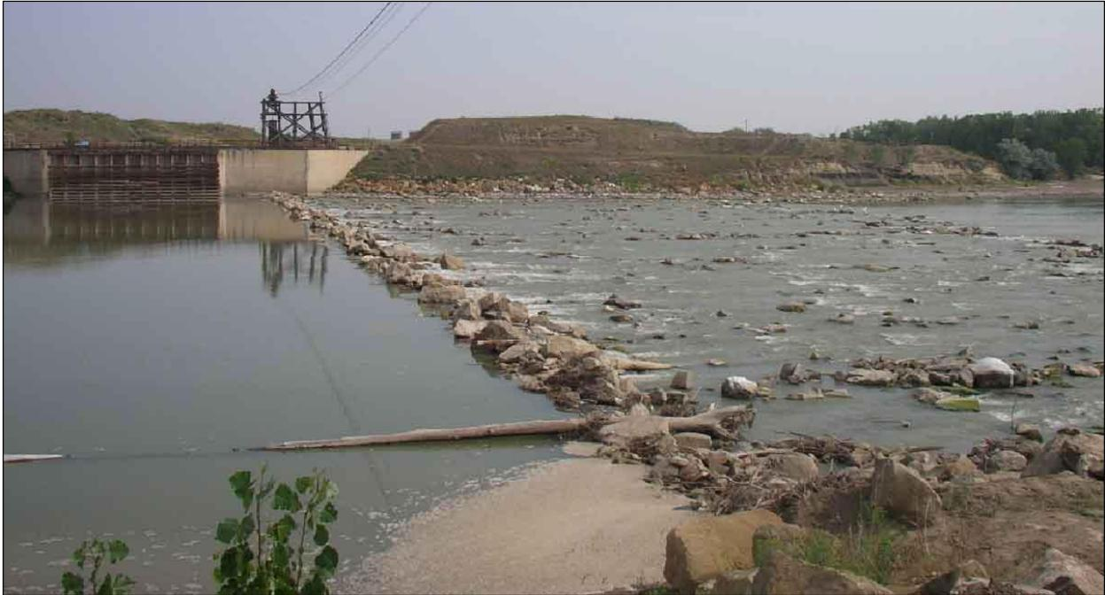
Figure 4-30 Intake Diversion Dam showing old headworks (USBOR)
